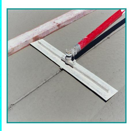
Early hand grooving forces the coarse aggregate particles away from the location of the groove and establishes the layer of mortar paste that must fill all defects in subsequent finishing passes.
