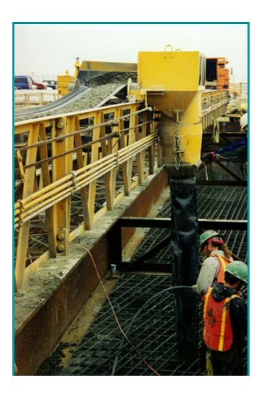
To Avoid Segregation-Limit Unconfined freefall of concrete to 5 ft. max.
