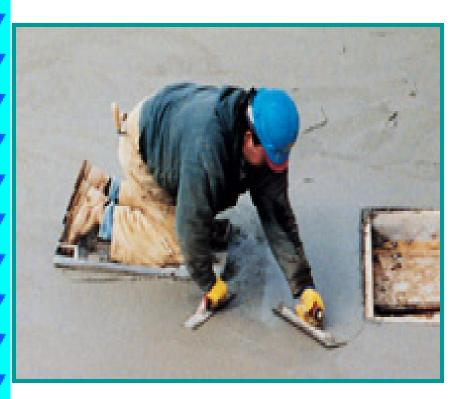
Creates smooth, hard, dense surface Exterior concrete should not be troweled because:
