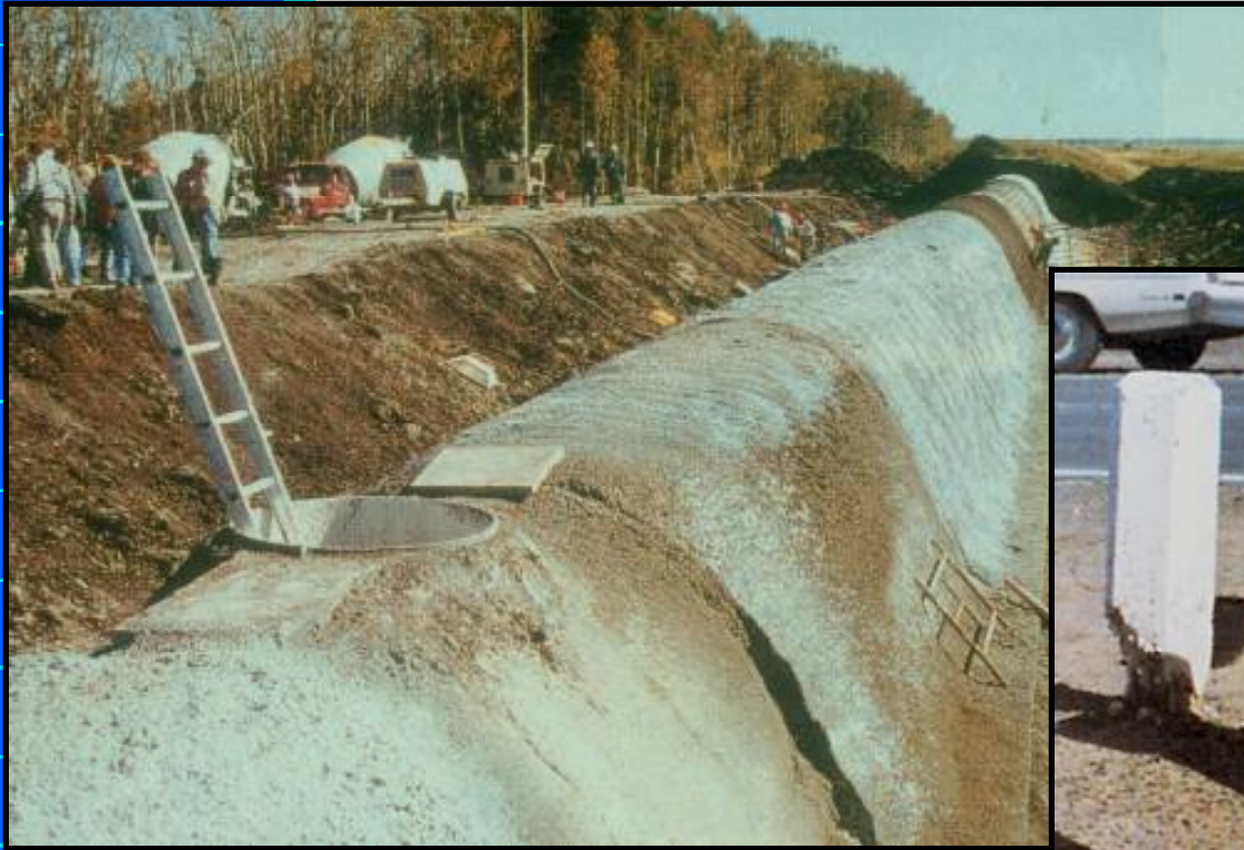
Examples of Sulfate Attack in Concrete Structures
