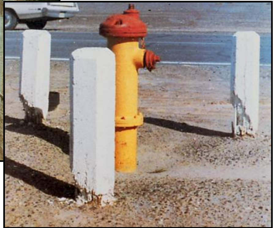
Examples of Sulfate Attack in Concrete Structures
