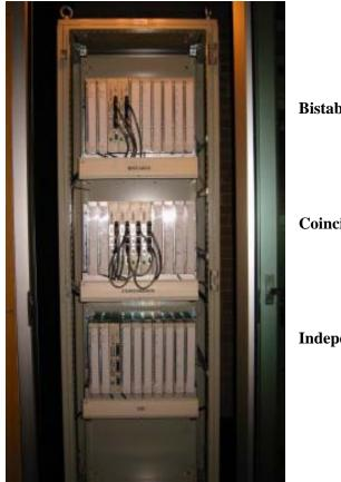
Figure 2-54 Westinghouse Common Q (AC160) PLC Rack
