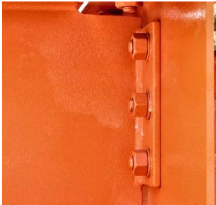
Shear End Plate Connection
