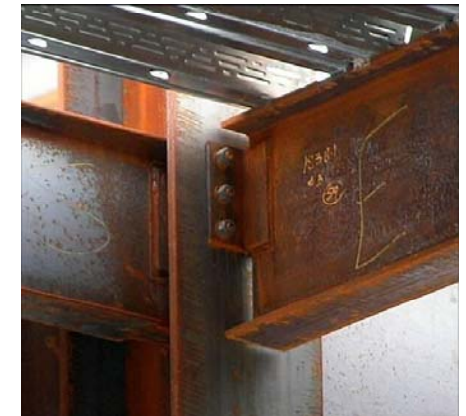
Double Angle Connection
