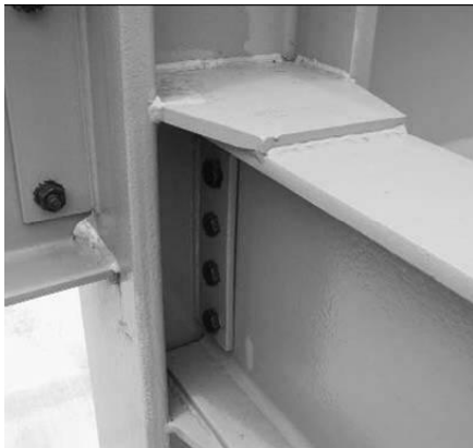
Welded Flange Plate Connection
