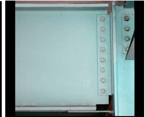
Partially-Restrained (PR) Connections
