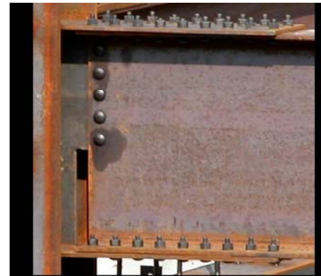
Fully-Restrained (FR) Connections
