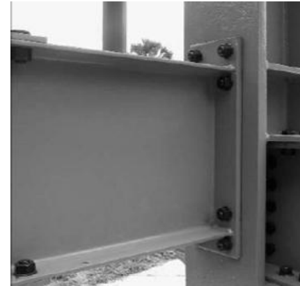
Bolted Extended End-Plate Connection
