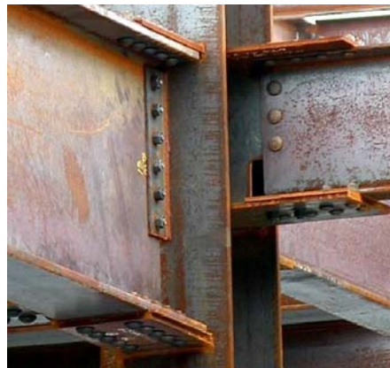
Bolted Flange Plate Connection
