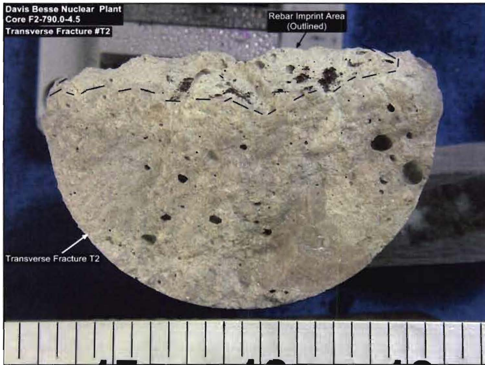
Figure A 5: Rebar Rib Groove Imprints (Core F2-790.0-4.5)
