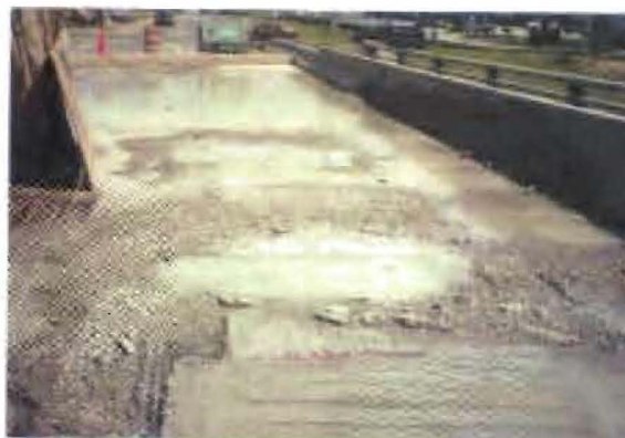
Figure 2: Note the straw bails covered with burlap at the end of the bridge to filter waste water.
