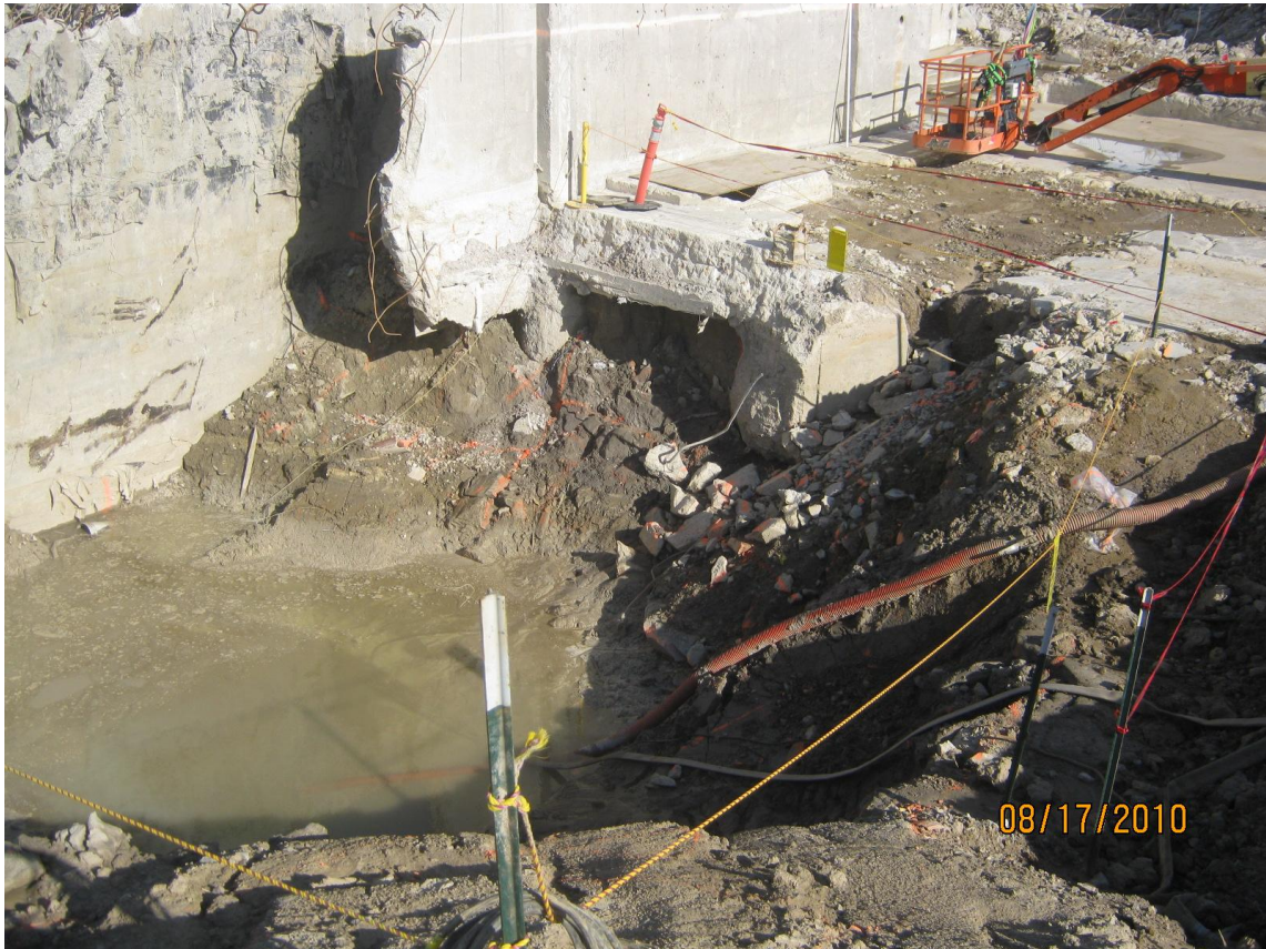
Exhibit 8, Excavation of WHB Evaporator Pit (August 2010)
