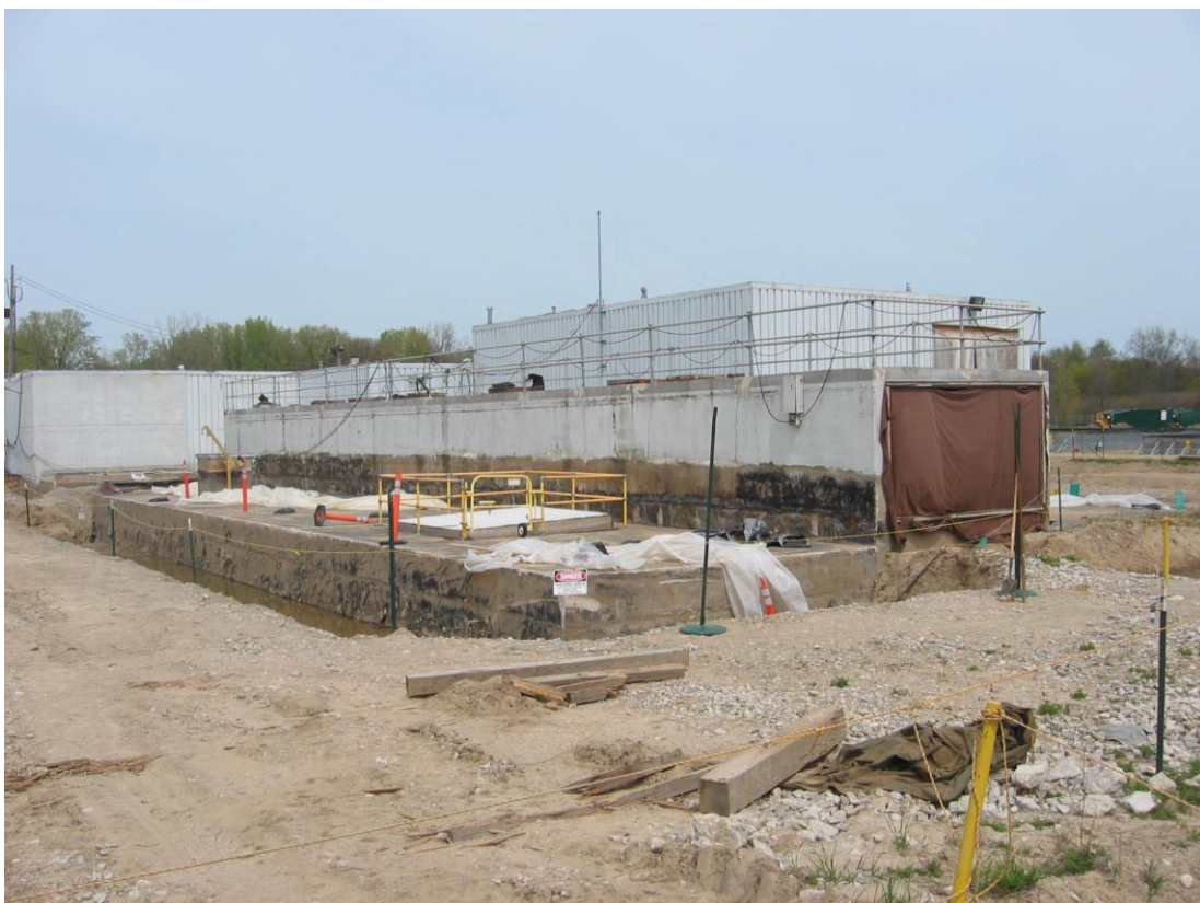
Exhibit 9, HRA After Overburden Removed Prior to Excavation (February 2010)
