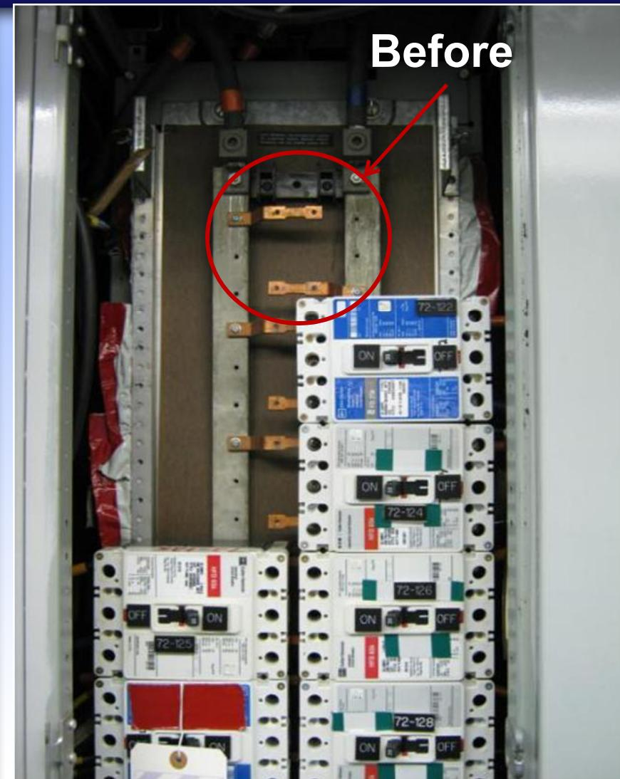
*A reactor scram occurred when a worker was performing maintenance activities on an electrical panel. The highlighted metal pieces have opposite charge, when they came into contact, they caused an electrical arc and loss of the bus.*
