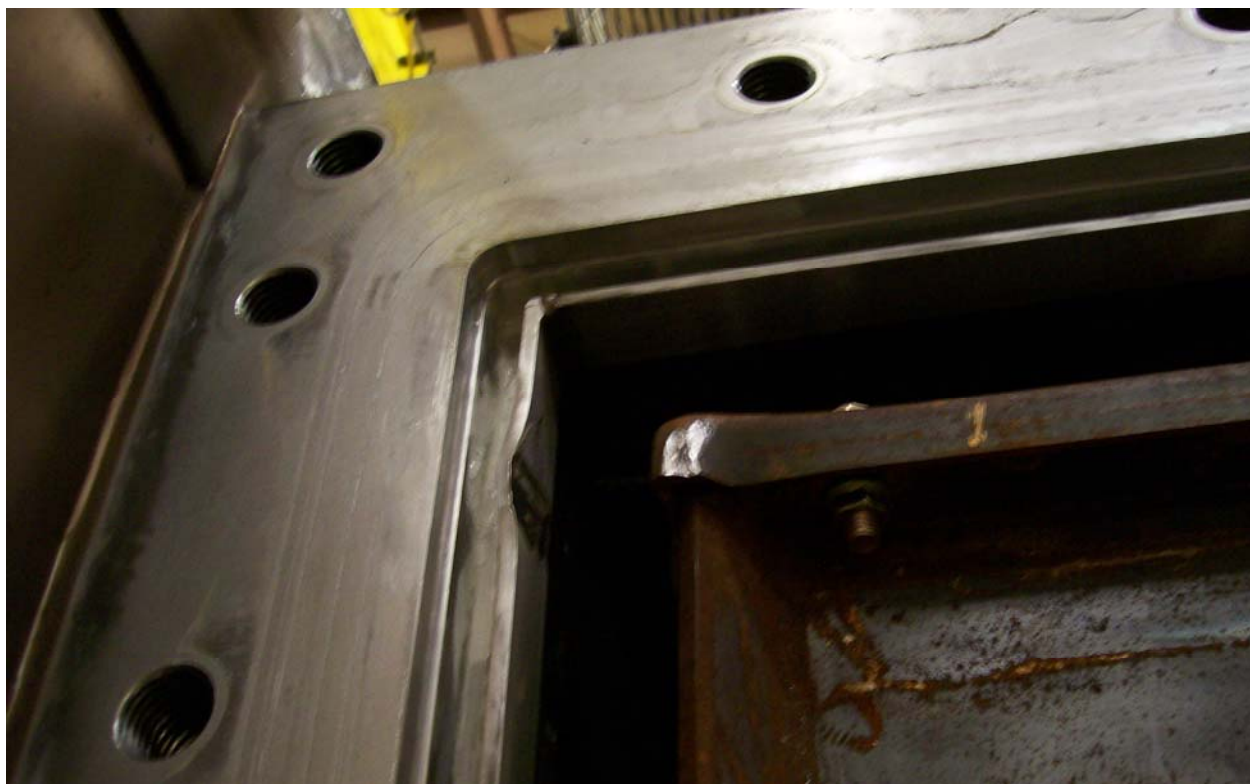
Figure 2.12.6-19 – Dent in Debris Shield Receptacle Caused by SLB2
