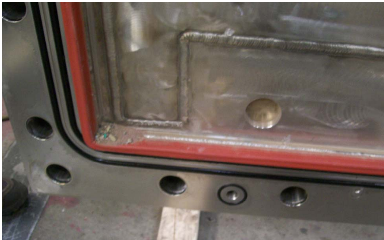
Figure 2.12.6-17 – Debris and Debris Shield (red) Upon Closure Lid Removal
