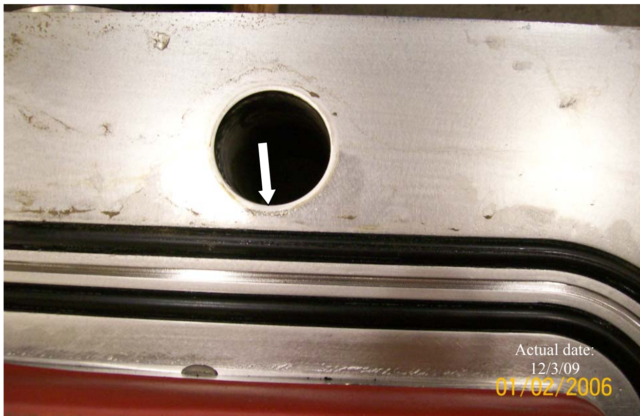
Figure 2.12.6-18 – Galling on Flange Around Closure Bolt Holes
