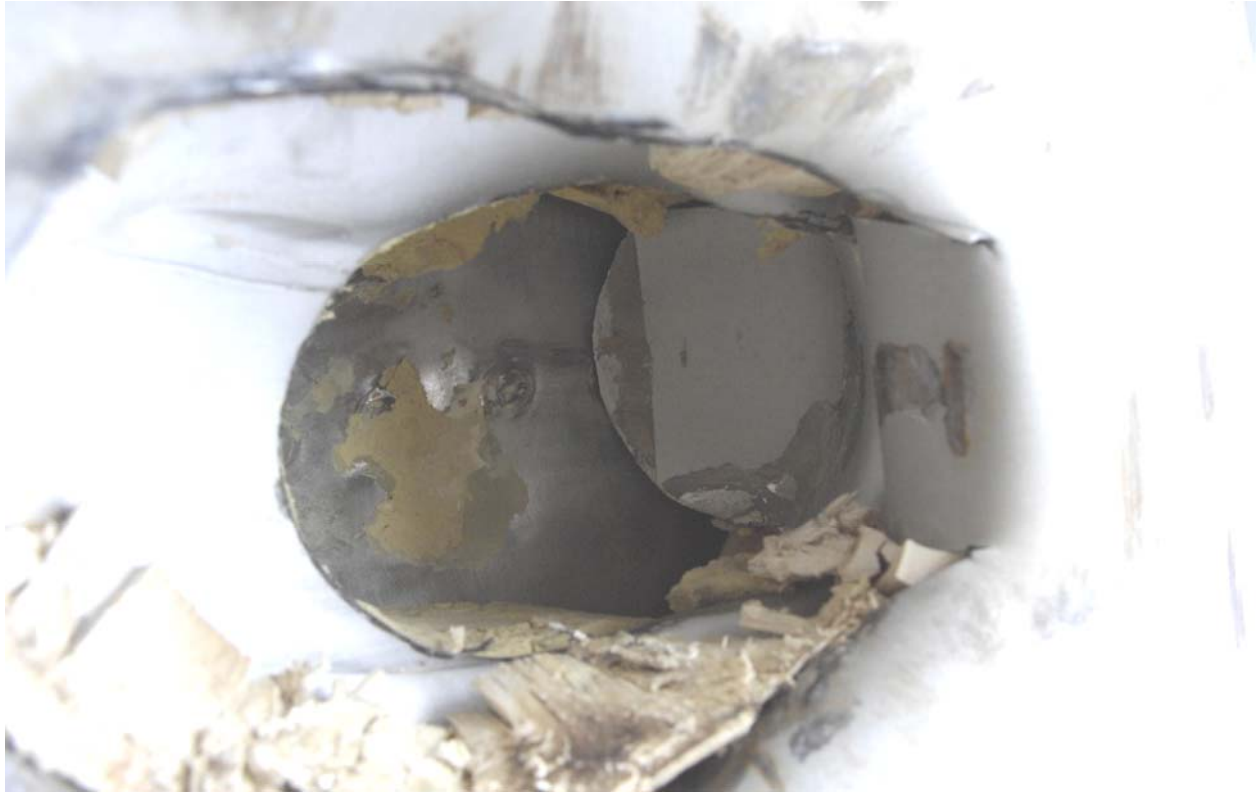
Figure 2.12.3-26 – Test LP1, Close-up of Damage. Bottom of Hole is CSA Outer Structural Sheet
