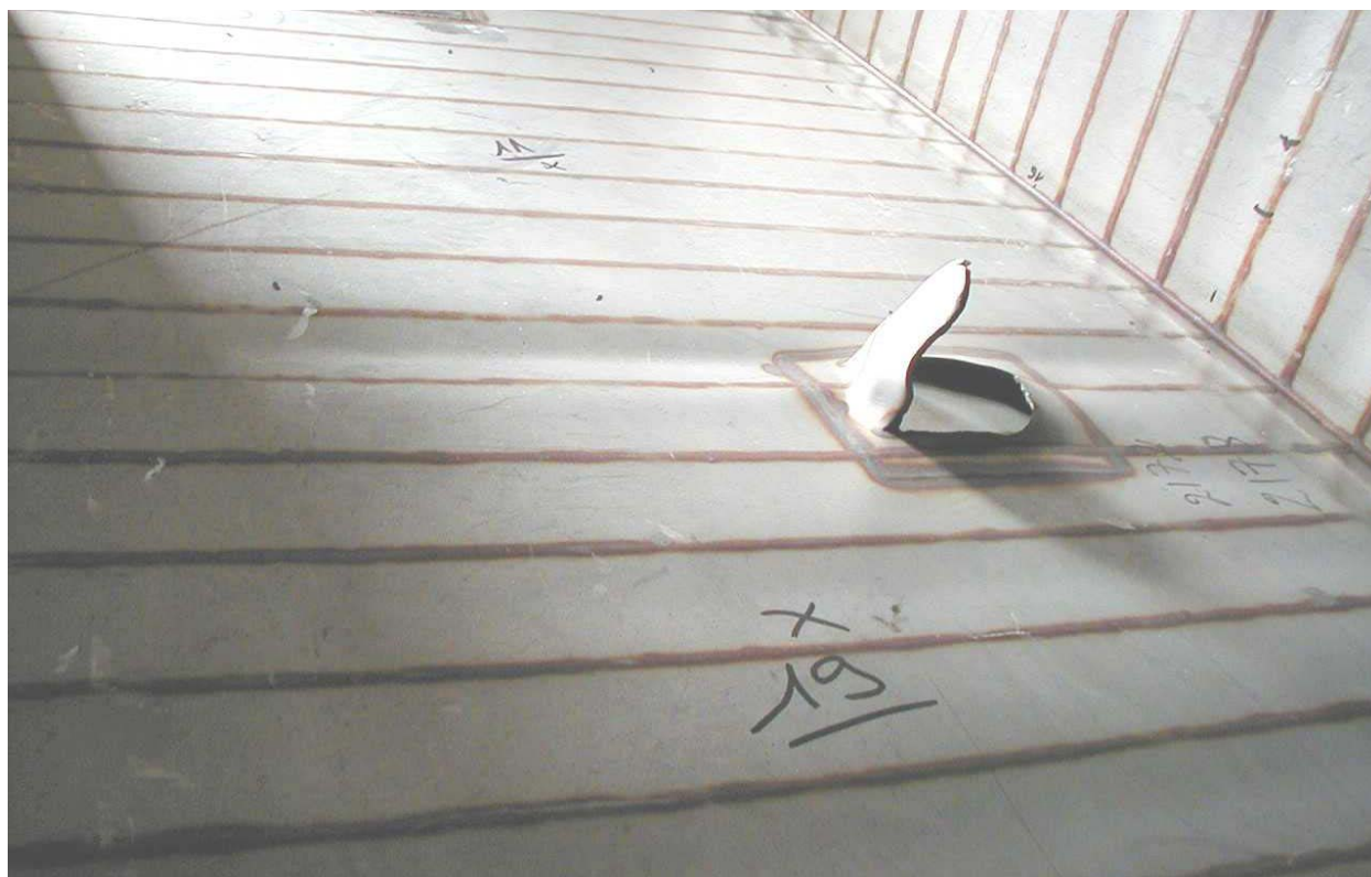
Figure 2.12.1-20 – Puncture Drop Test F5: View of Internal Damage (with Welded Patch)
