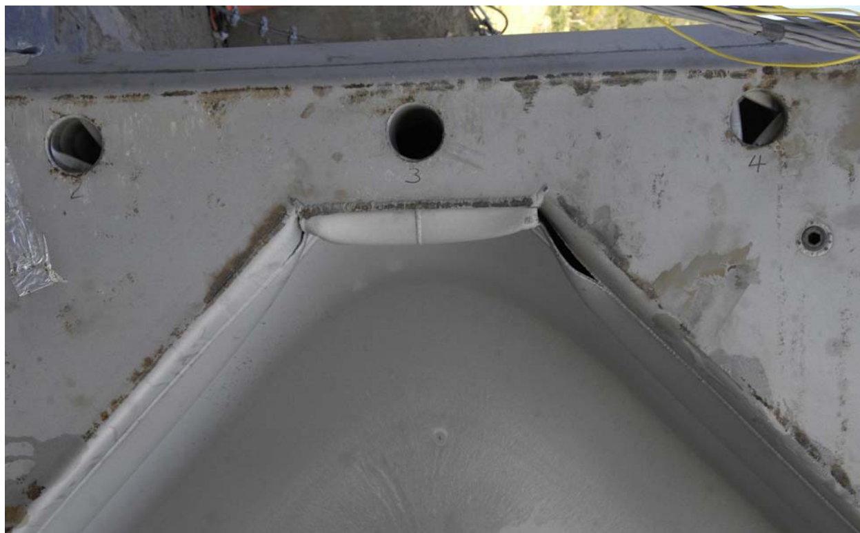
Figure 2.12.3-11 – Test LD2, Typical Torn Welds on Overpack Cover
