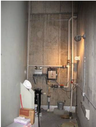
Photograph 24 10K Tank Room
