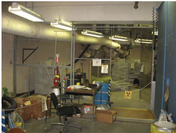
Photograph 59 Main Floor Neutron Level
