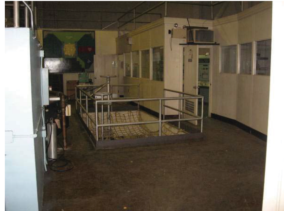
Photograph 41 Main Floor Control Deck
