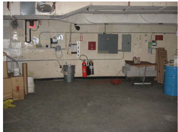
Photograph 63 Main Floor Neutron Level
