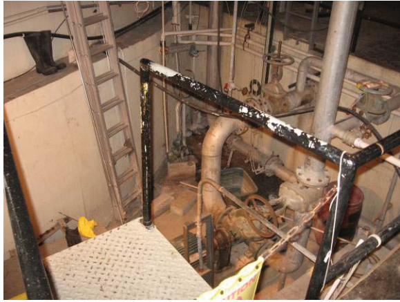
Photograph 30 Room N03 1K Tank Pit
