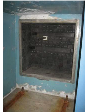
Photograph 67 Thermal Column
