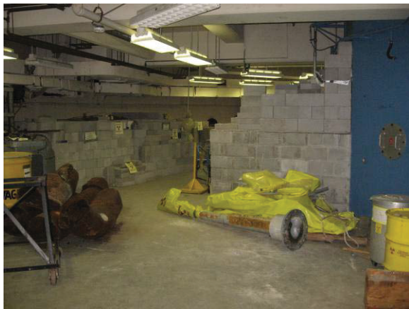
Photograph 60 Main Floor Neutron Level
