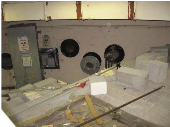
Photograph 65 Beam Port Storage Tubes
