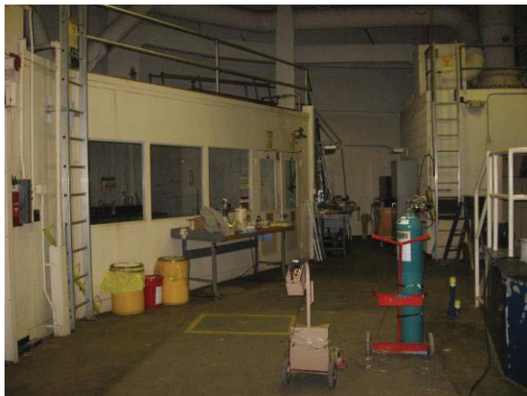
Photograph 40 Main Floor Control Deck
