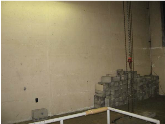
Photograph 2 OTB (Vertical Accelerator Room)
