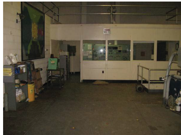
Photograph 43 Main Floor Control Deck
