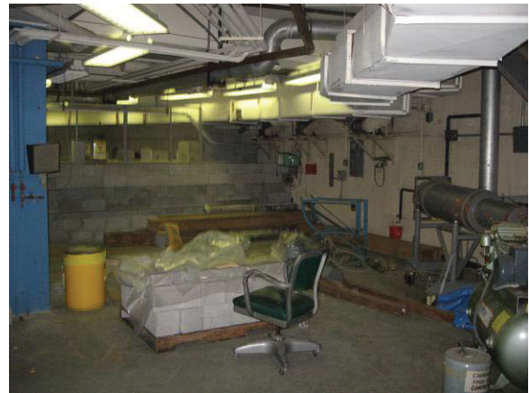
Photograph 62 Main Floor Neutron Level
