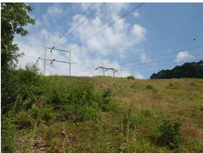
Photograph 10. Area 13 East: Disturbed Transmission Corridor on Steep Slope, Facing Northeast
