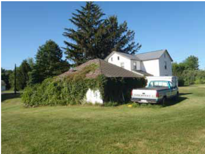
Photograph 15. Area 14: Garage and House, Facing Southwest
