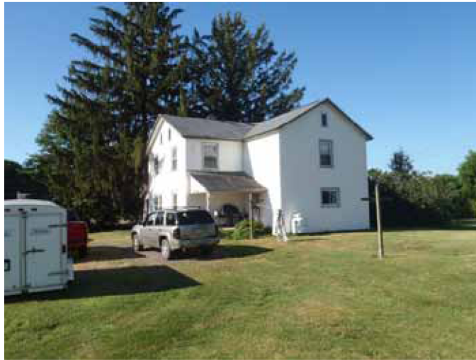
Photograph 14. Area 14: Rear Façade of House, Facing Southwest
