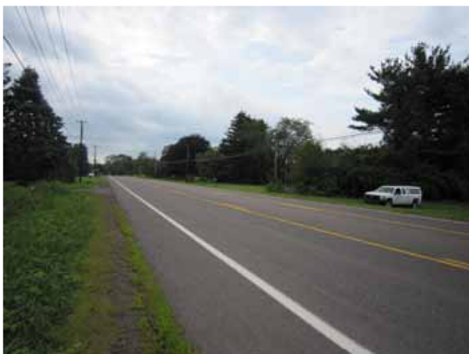
Photograph 8. Area 12: Test Area within US Route 11 Right-of-Way, Facing Northwest
