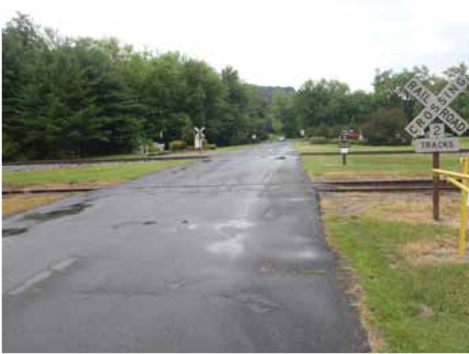
Photograph 5. Area 1: Paved Access Road Crossing SSES Rail Spur and former Bloomsburg Division of the Delaware, Lackawanna & Western Railroad (155053/GAI-11), Facing East
