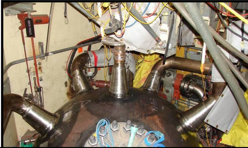
Pressurizer Nozzle Structural Overlays ( dia. ~100mm, ~200mm, ~350mm )
