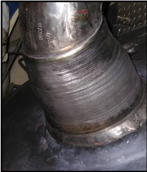
In-process 52M Overlay on Pressurizer Safety Nozzle
