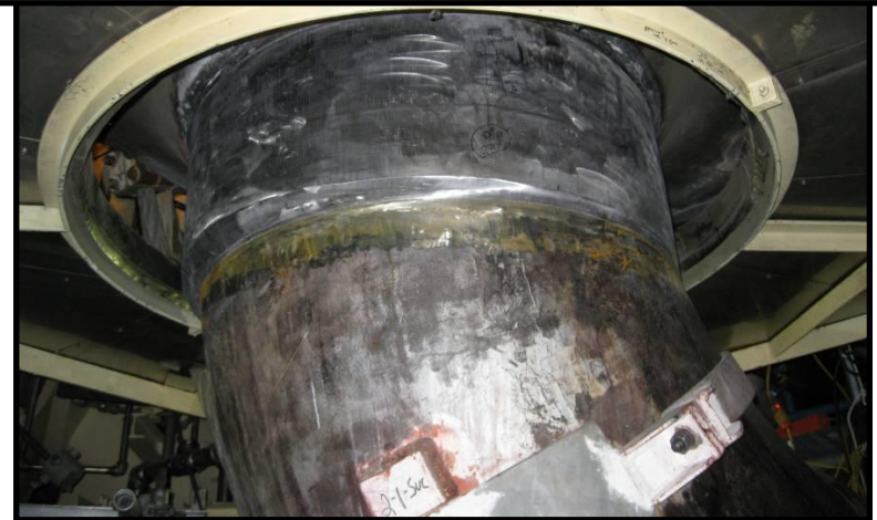
Reactor Coolant Pump Suction Nozzle Optimized Overlay ( dia ~850mm )
