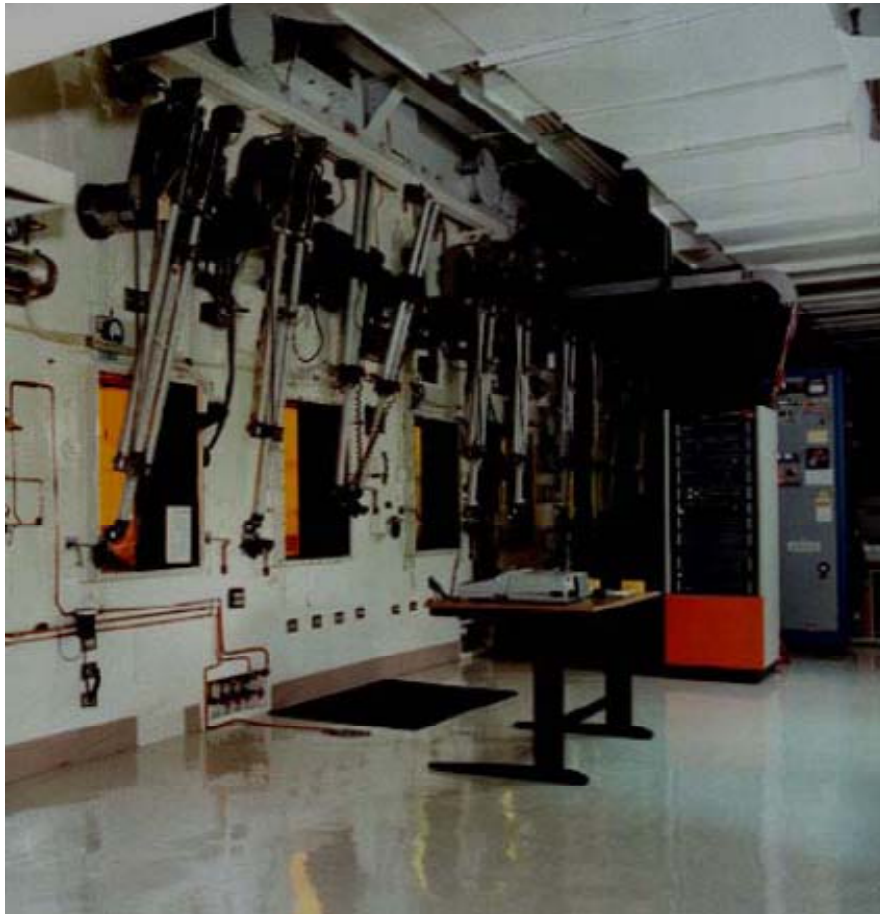
Special welding cell at ORNL
