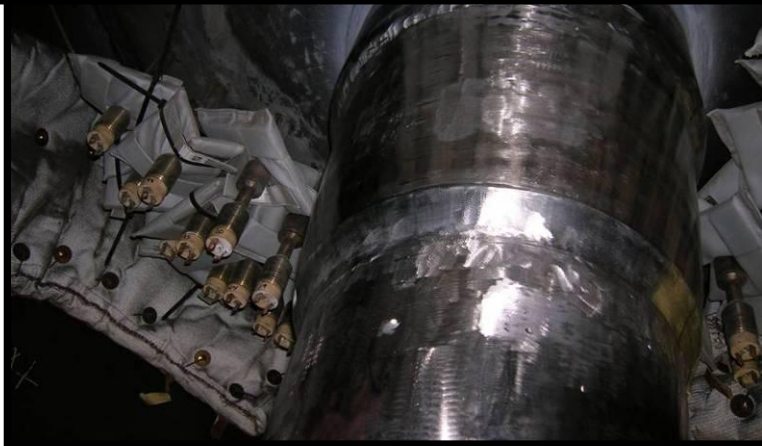
Pressurizer Nozzle Structural Overlays ( dia. ~100mm, ~200mm, ~350mm )
