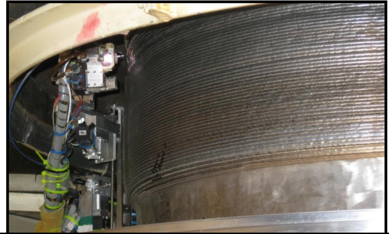
Reactor Coolant Pump Suction Nozzle Optimized Overlay ( dia ~850mm )
