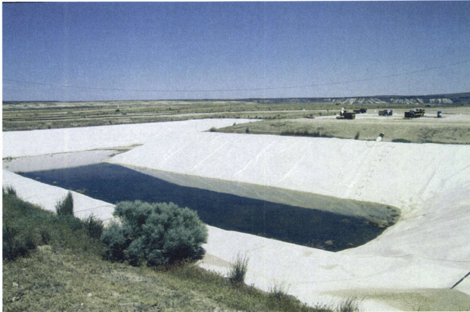
Figure 1.11 :Evaporative Surface Impoundment
