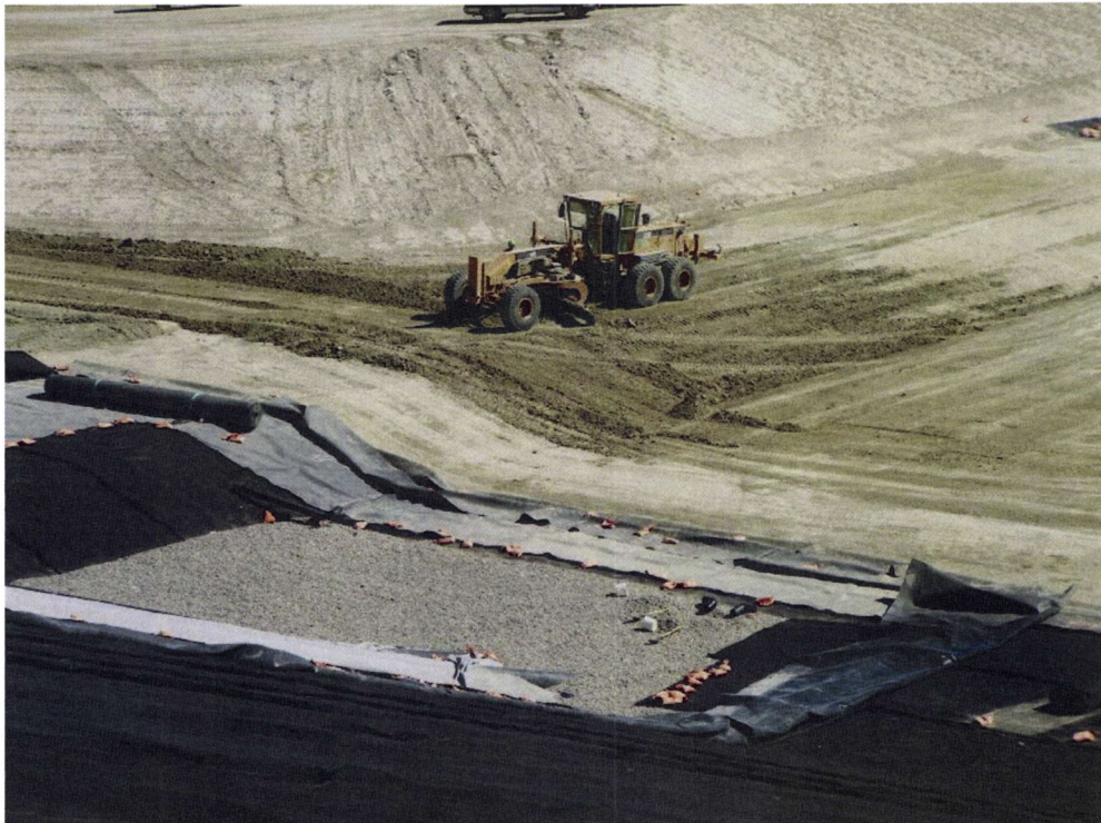
Figure 1.9 :Cell 15 Liner Installation
