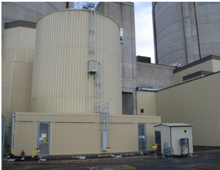
Unit 1 – Looking East
