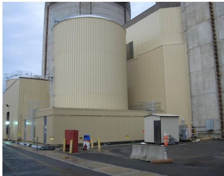
Unit 2 – Looking North
