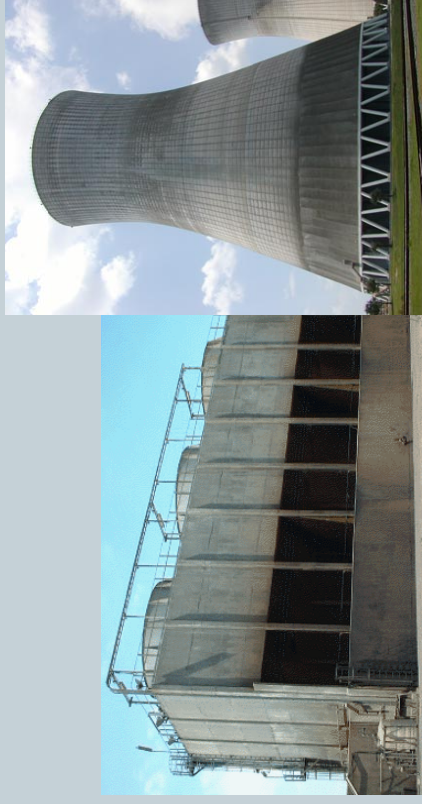
Mechanical Draft Cooling Towers (Source: wetcooling.com 2011)
