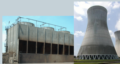
Mechanical Draft Cooling Towers (Source: wetcooling.com 2011)
