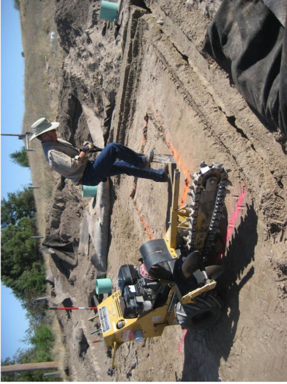
Fig. A.29. Installation of SDRI seating trenches.
