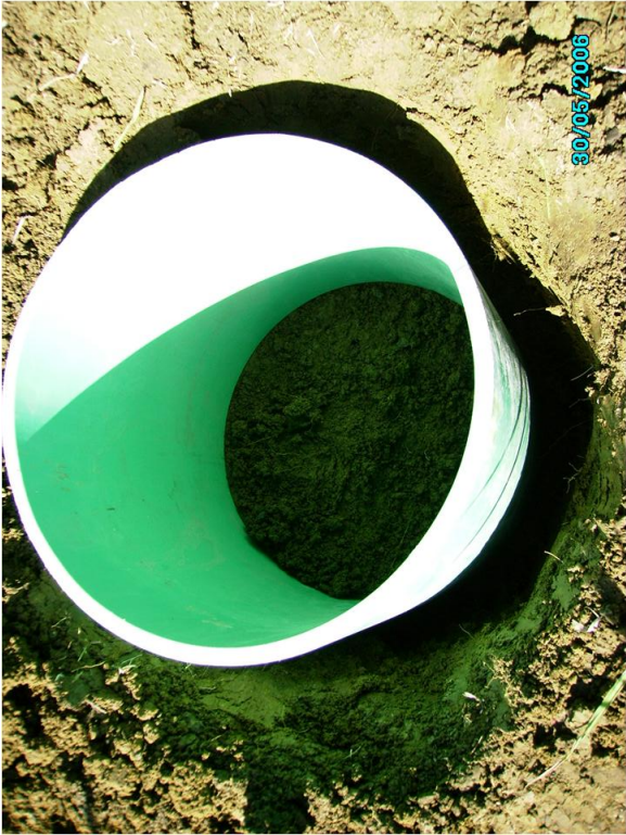
Fig. A.43. Installing TSB, rough bottom to avoid smearing.
