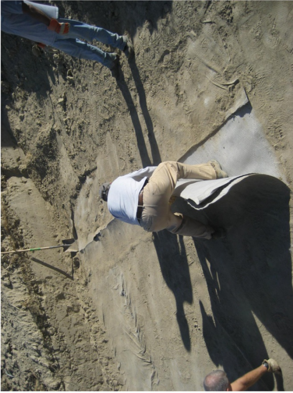
Fig A.5. Sampling GDL in section with composite barrier.
