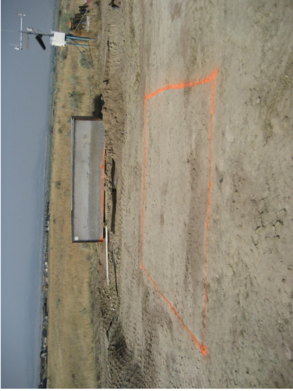
Fig. A.11. Cover soil removed prior to SDR1 installation.
