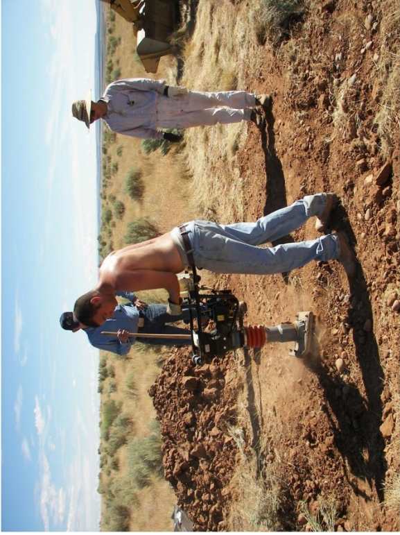
Fig. A.97. Re-compacting soil after sampling.
