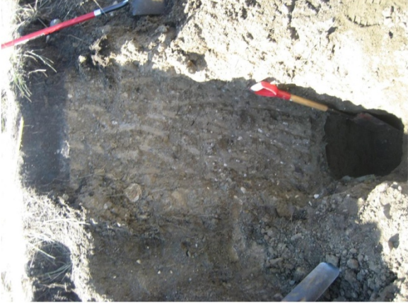
Fig. A.75. Thicker CCL (5 ft), desiccation and roots visible throughout profile.
