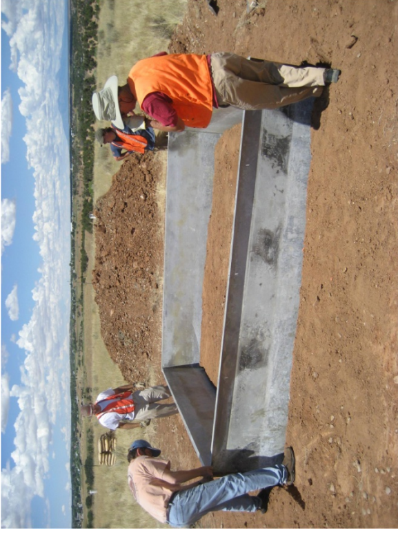
Fig. A.85. Setting SDR1 in trenches.
