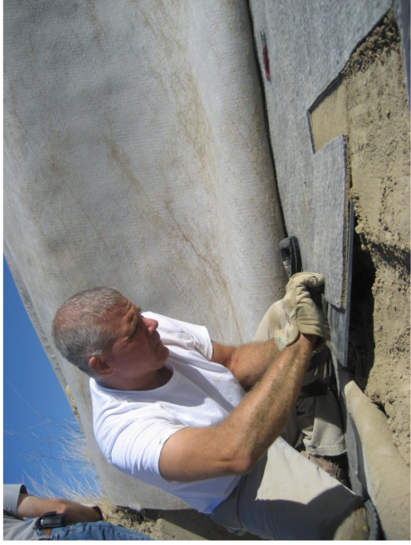
Fig A.6. Constructed defect in GM.
