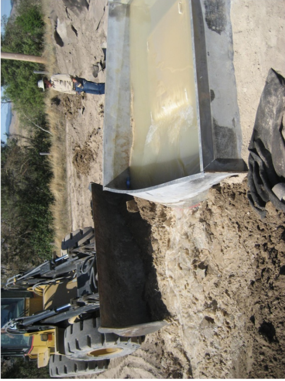
Fig. A.37. Water removal from completed SDRI.
