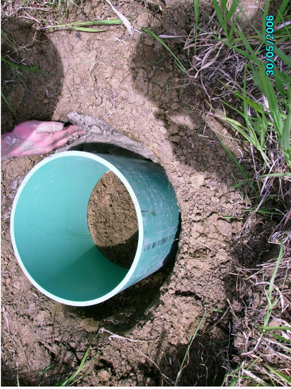
Fig. A.44. Grouting TSB with bentonite paste.
