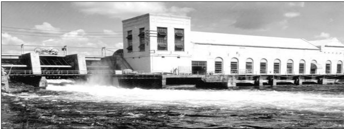
Figure 13. 1955 photograph of the Dunnellon Dam and Hydro-Electric Power Plant. Source: Florida Center for Instructional Technology, University of South Florida.
