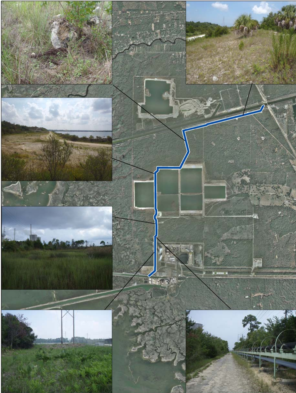
Figure 19. Counterclockwise from top left: dragline for land clearing and limerock boulder; looking east along access road on the north side of the Holcim property; looking southeast toward the CREC facility; looking north from CREC toward the Holcim property; looking south along the access road and Holcim conveyor system; looking east along the berm adjacent to the barge canal.
