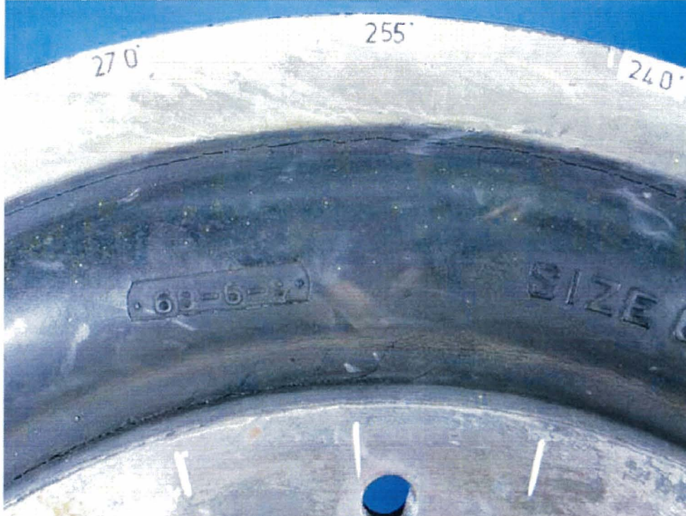
Figure 4 Circumferential crack in EDG flexible coupling
