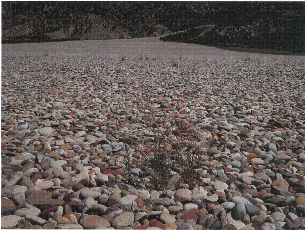
RFL 8/2011. PL-3. View (to northeast) of isolated shallow-rooted weeds on cell.
