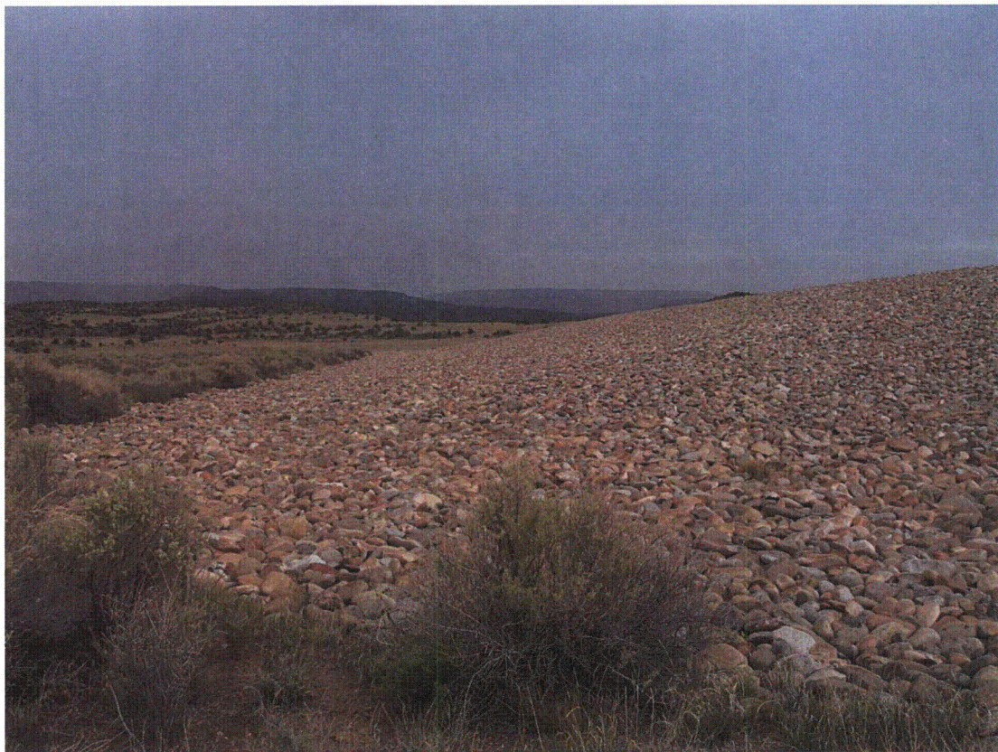
SRK 7/2011. PL- 3. Southeast face of cell.
