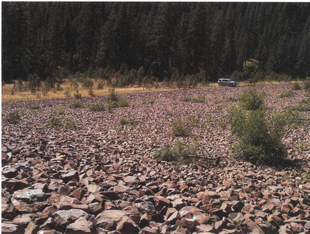
LOW 7/2011. PL-2. View of riprap on southwest slope (cut trees in foreground).
