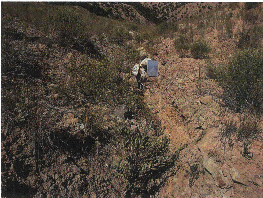
RFL 8/2011. PL-4. New gully erosion (4 to 6 inches) in upper section of inceptor trench.
