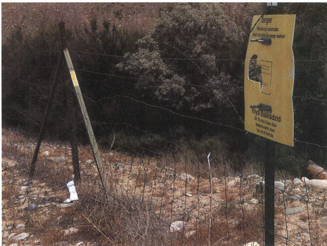
SHP 6/2011. PL-4. Broken fence wire and warning sign.
