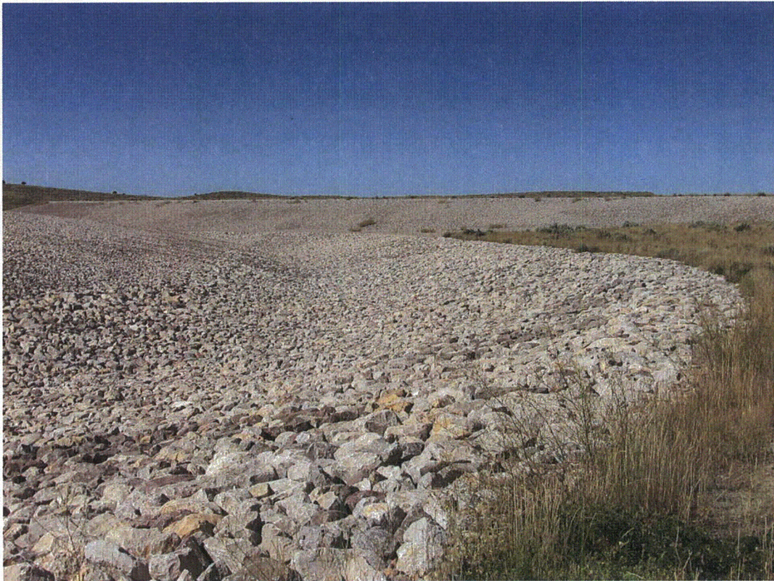
MAY 8/2011. PL-6. Diversion Channel No. 1; rock-covered slope west of cell in background.
