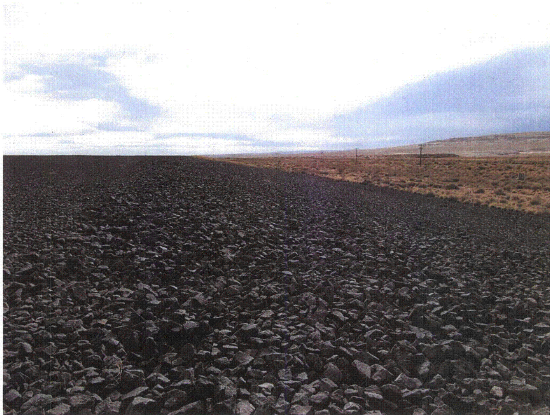
TUB 4/2011. PL-2. South side slope of the disposal cell cover.
