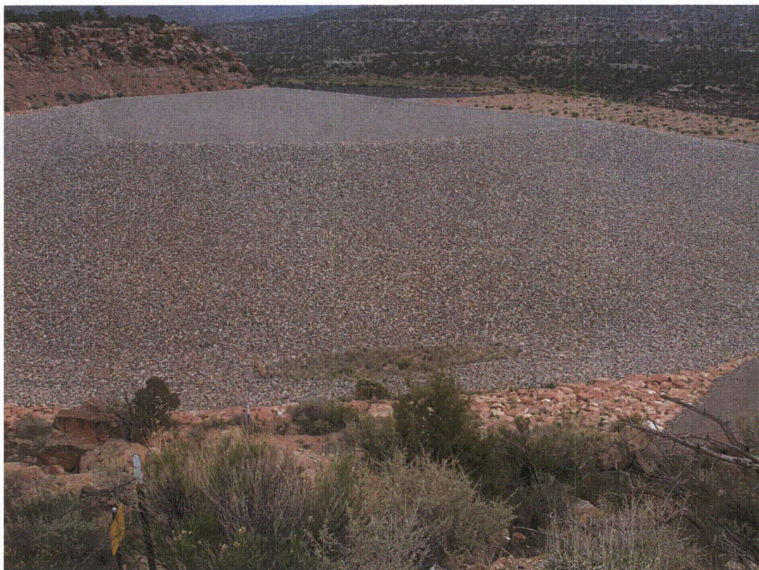
NAT 5/2011. PL-1. Top of disposal cell, view to southeast.
