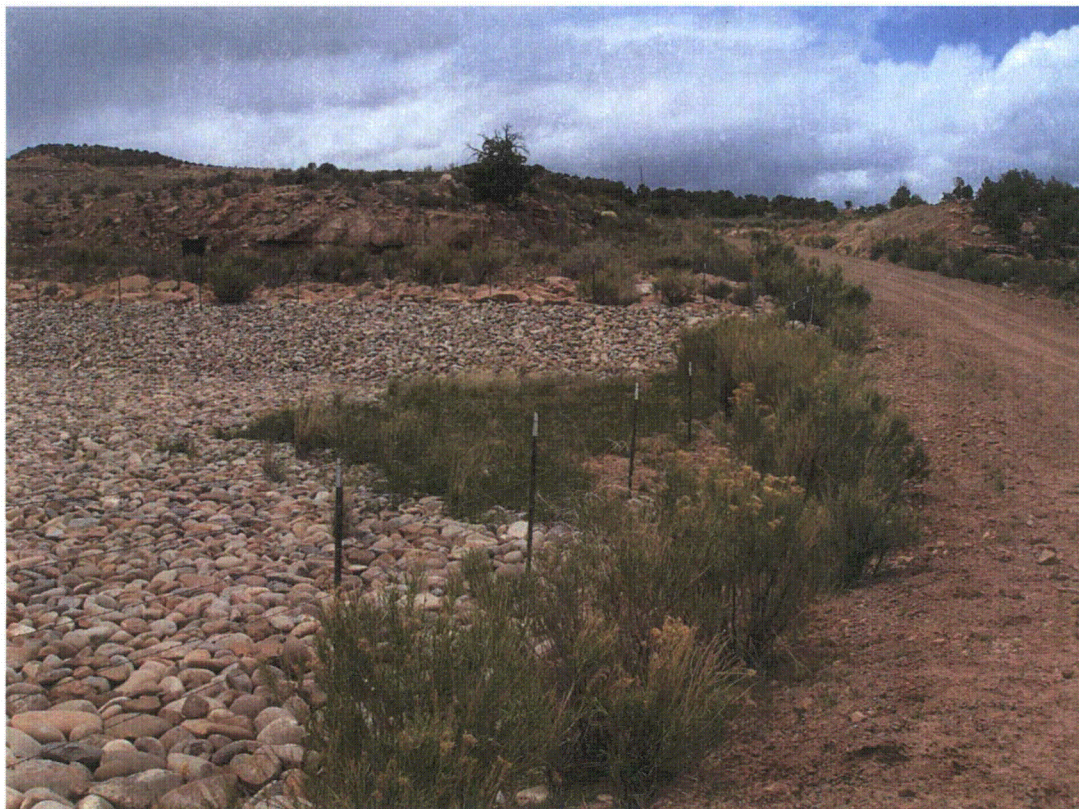
NAT 5/2011. PL-3. View of interceptor channel area from Country road (view to northwest).
