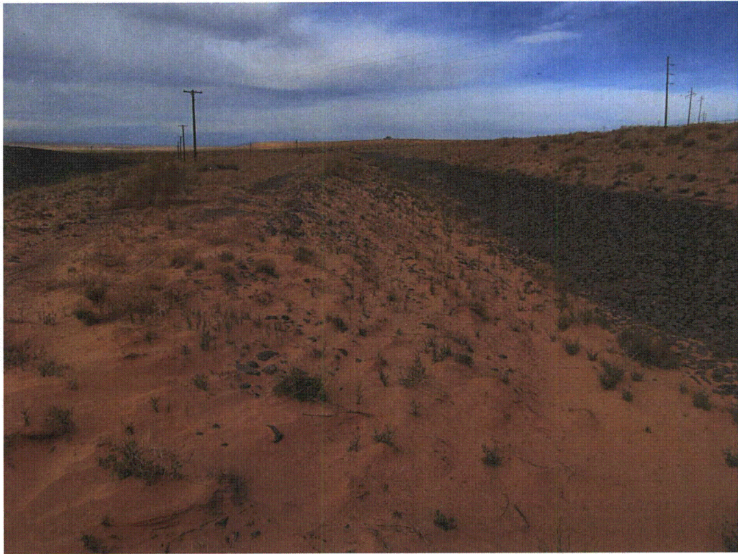
TUB 4/2011. PL-7. Windblown sand deposition on the south bank of the diversion channel.
