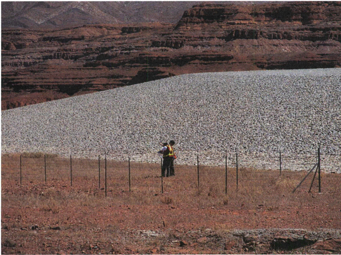
HAT 4/2011. PL-3. Inspectors along the northwest side of the disposal cell.
