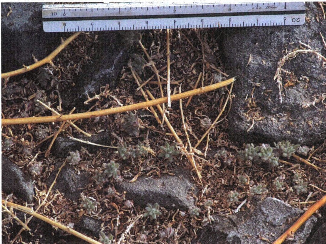
TUB 4/2011. PL-3. Windblown sand accumulation on the disposal cell cover.
