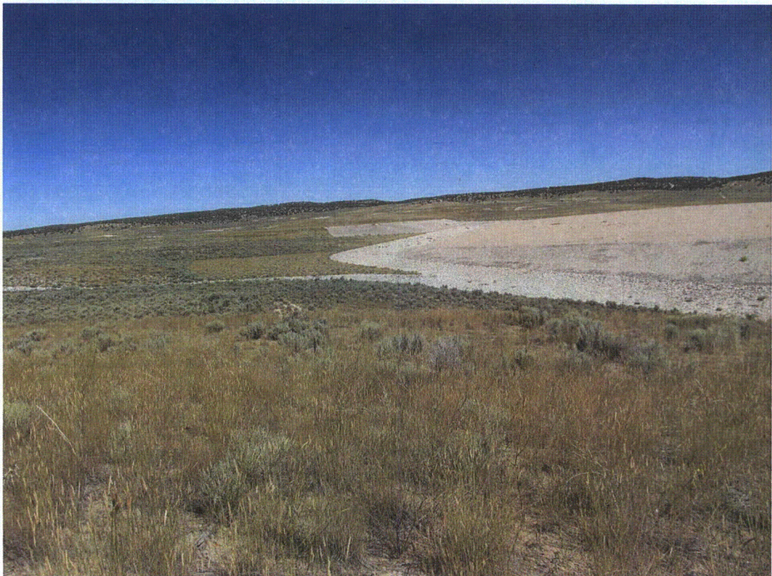
MAY 8/2011. PL-4. Western portion of the disposal cell and confluence of Diversion Channels Nos. 1 and 2.
