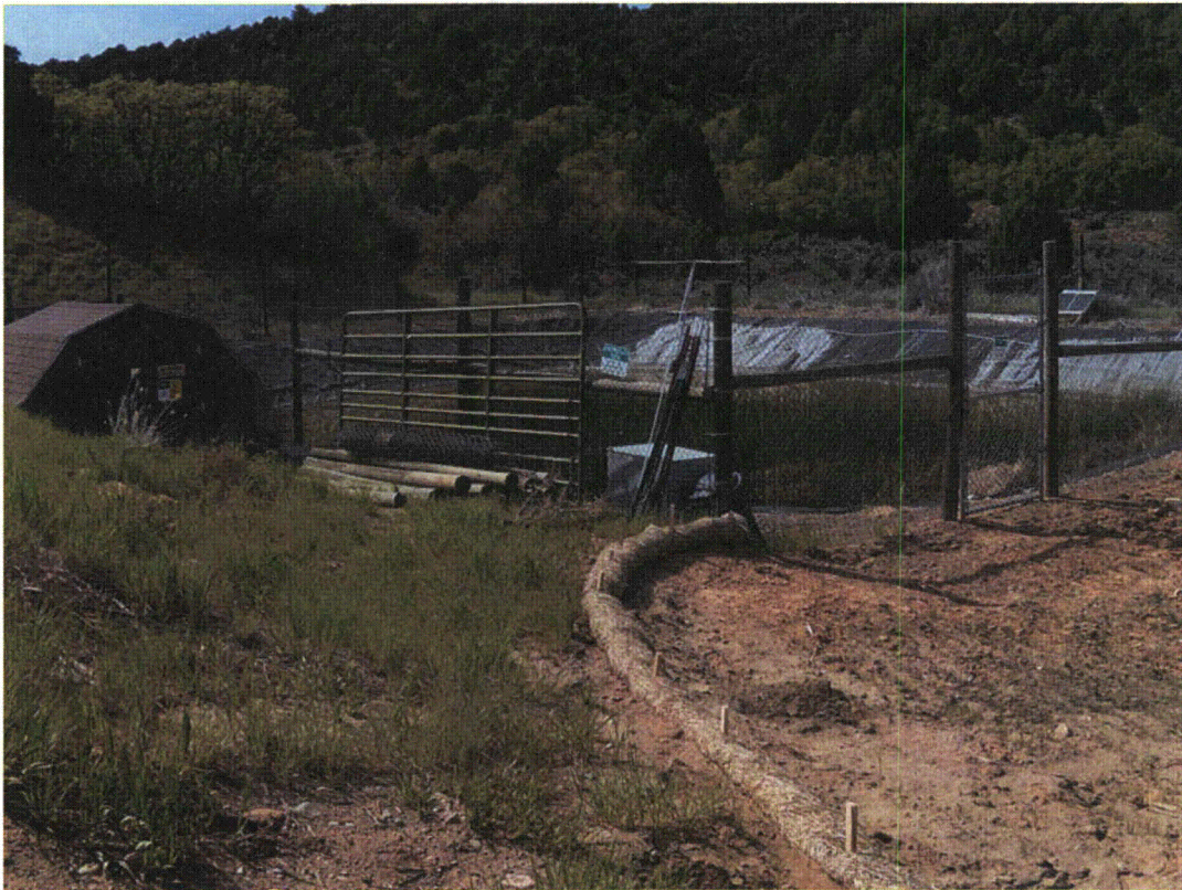
DUR 5/2011. PL-3. New fence around east side of retention pond area.
