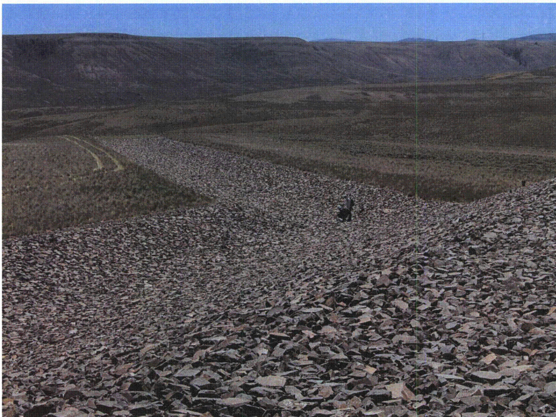
GUN 6/2011. PL-3. East diversion channel.
