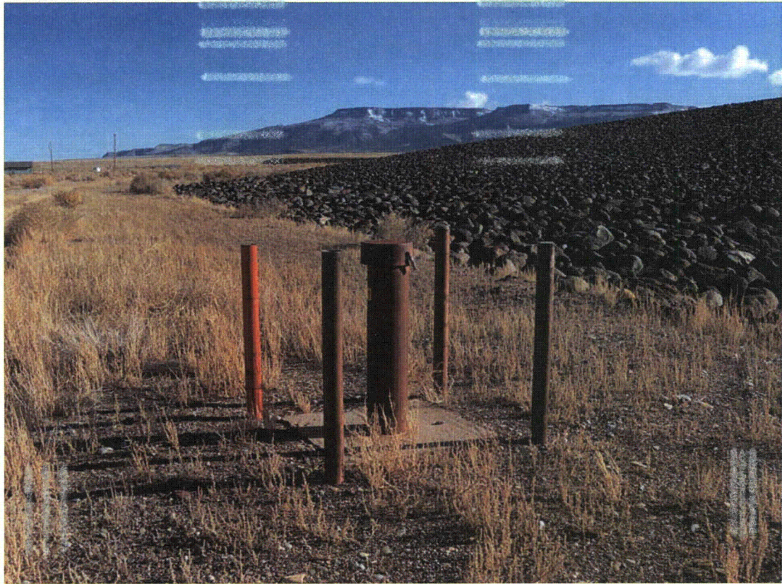
GRJ 3/2011. PL-1. Monitoring well 0731 near the northwest corner of the disposal cell.
