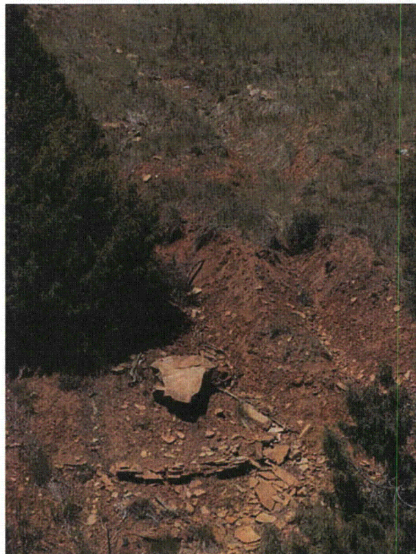
DUR 5/2011. PL-4. Headcuts of gullies below southwest corner of disposal cell; no change from 2009.
