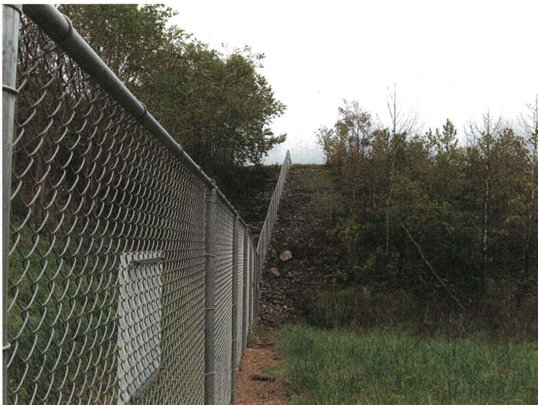
BUR 10/2011. PL-2. Vegetation cleared from perimeter fence.
