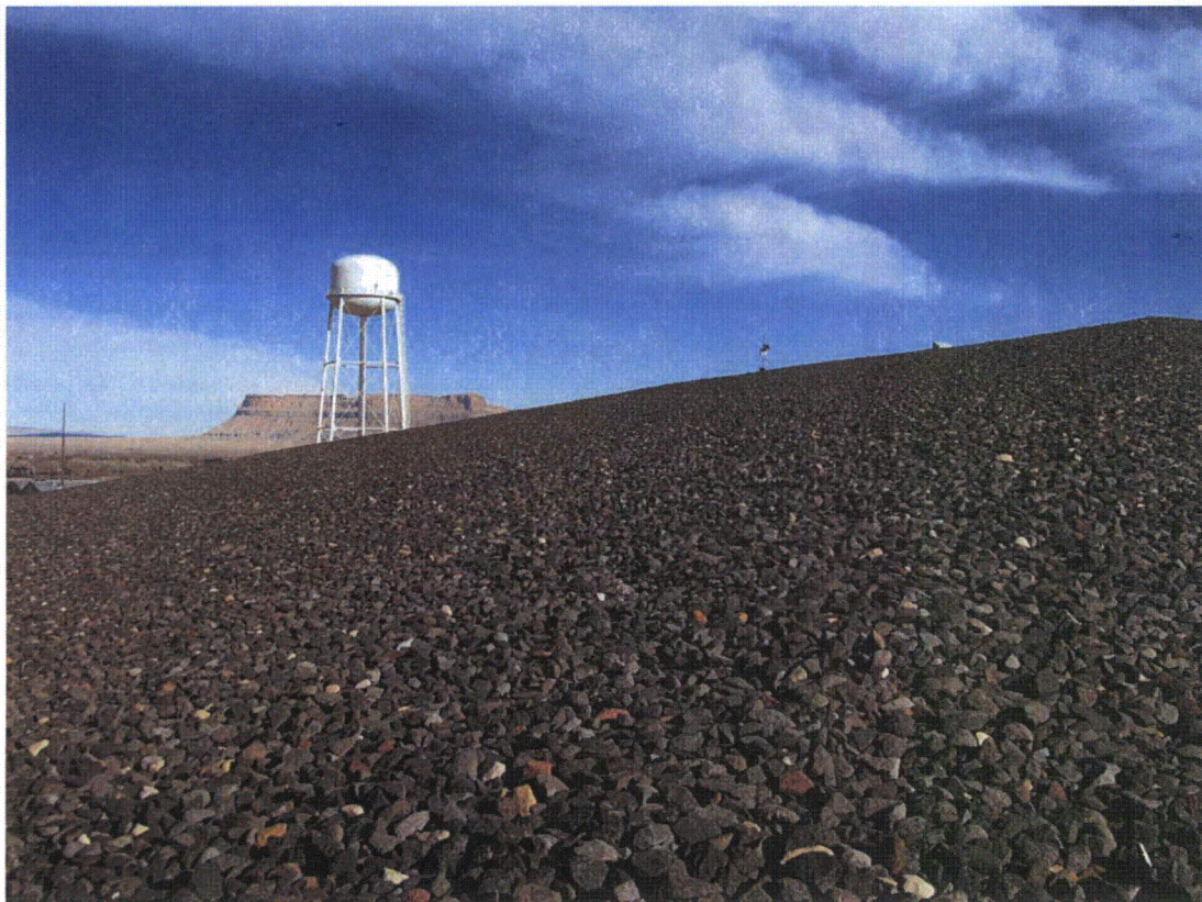
GRN 3/2011. PL-3. Southwest side slope of the disposal cell.
