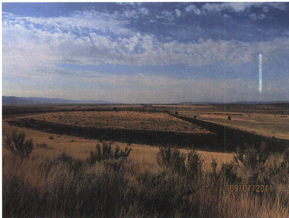
LKV 9/2011. PL-2. View from north site fence to south, showing cell top and side slopes.
