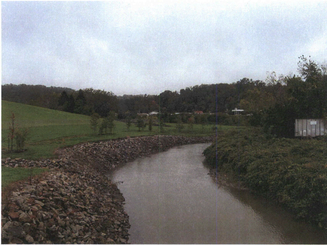
CAN 10/2011. PL-5. Contrast between riprap stream bank, where vegetation is managed, and non-riprap stream bank, where vegetation is not managed.
