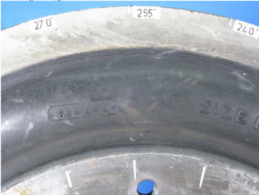
Figure 4 Circumferential crack in EDG flexible coupling
