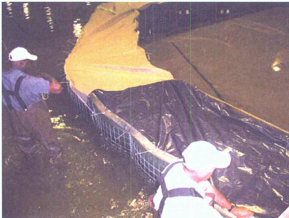
Figure 2-75. Securing with cable ties
