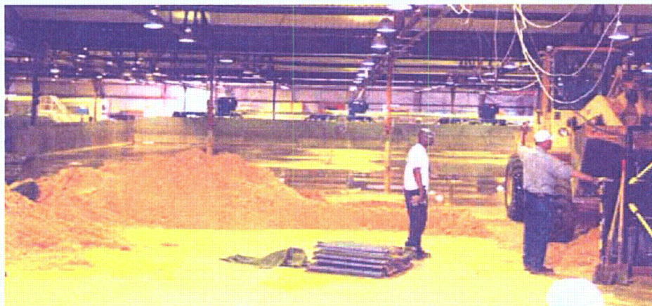
Figure 2-96. Stacked units ready for reuse
