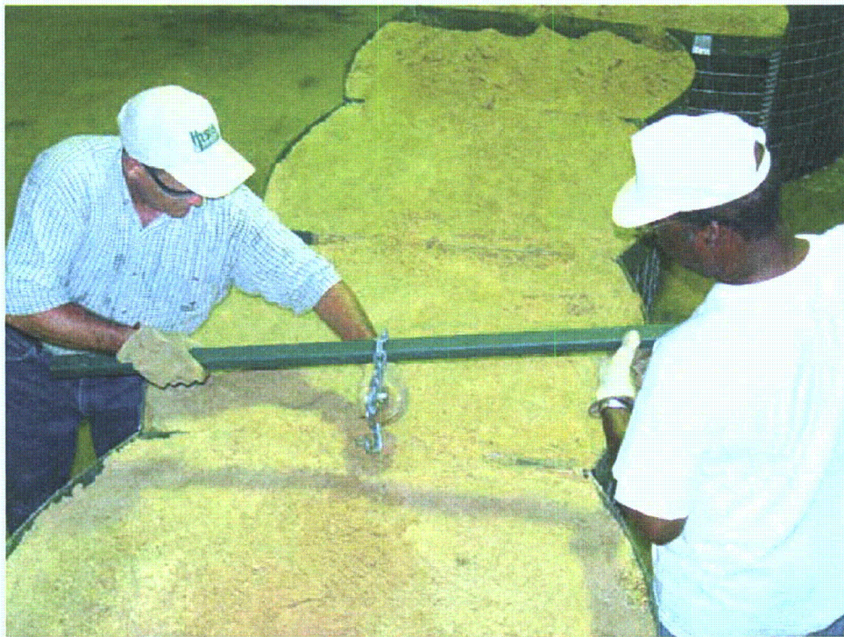
Figure 2-90. Preparing to remove center partition pin
