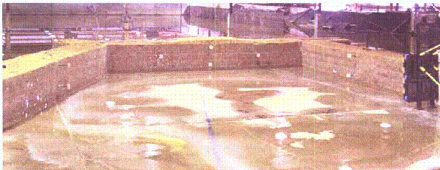
Figure 2-127. View from protected side
