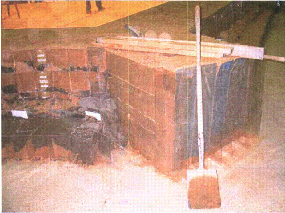
Figure 2-120. Completed sand and mixture fill viewed from pool side
