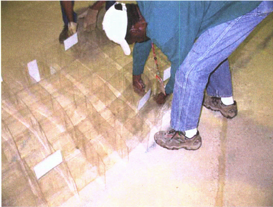
Figure 2-103. Connecting two grid units together
