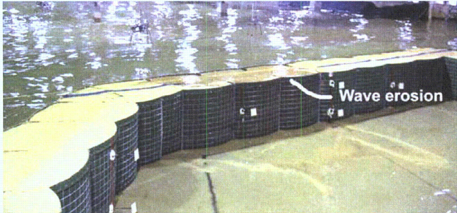
Figure 2-72. Center wall wave-induced erosion
