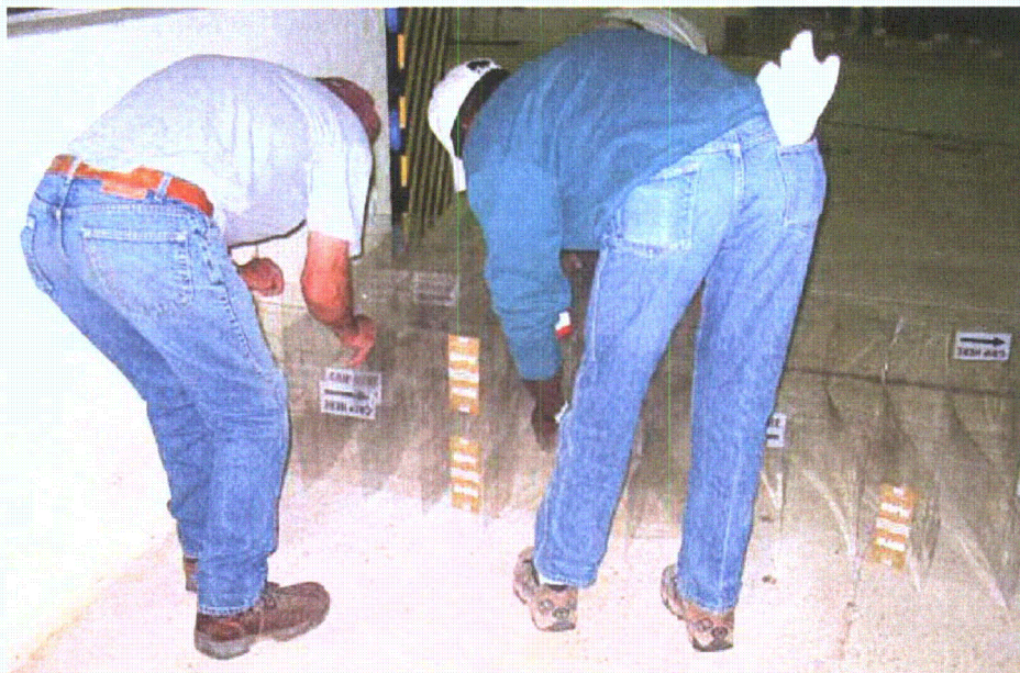
Figure 2-108. Beginning second grid layer from right concrete wall abutment
