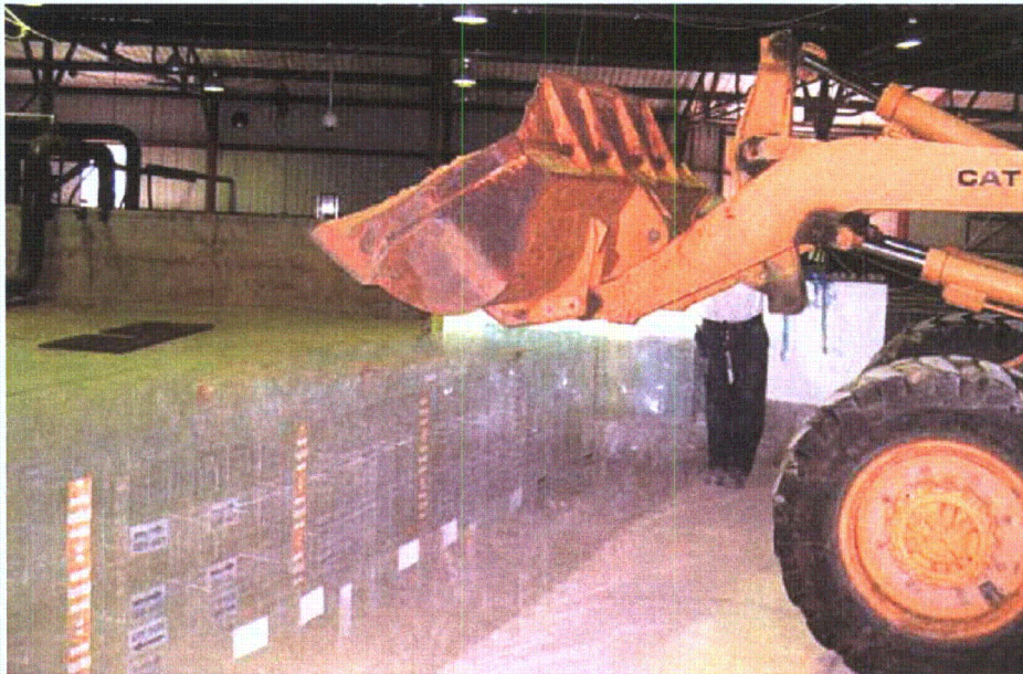
Figure 2-113. Begin sand fill on left wall
