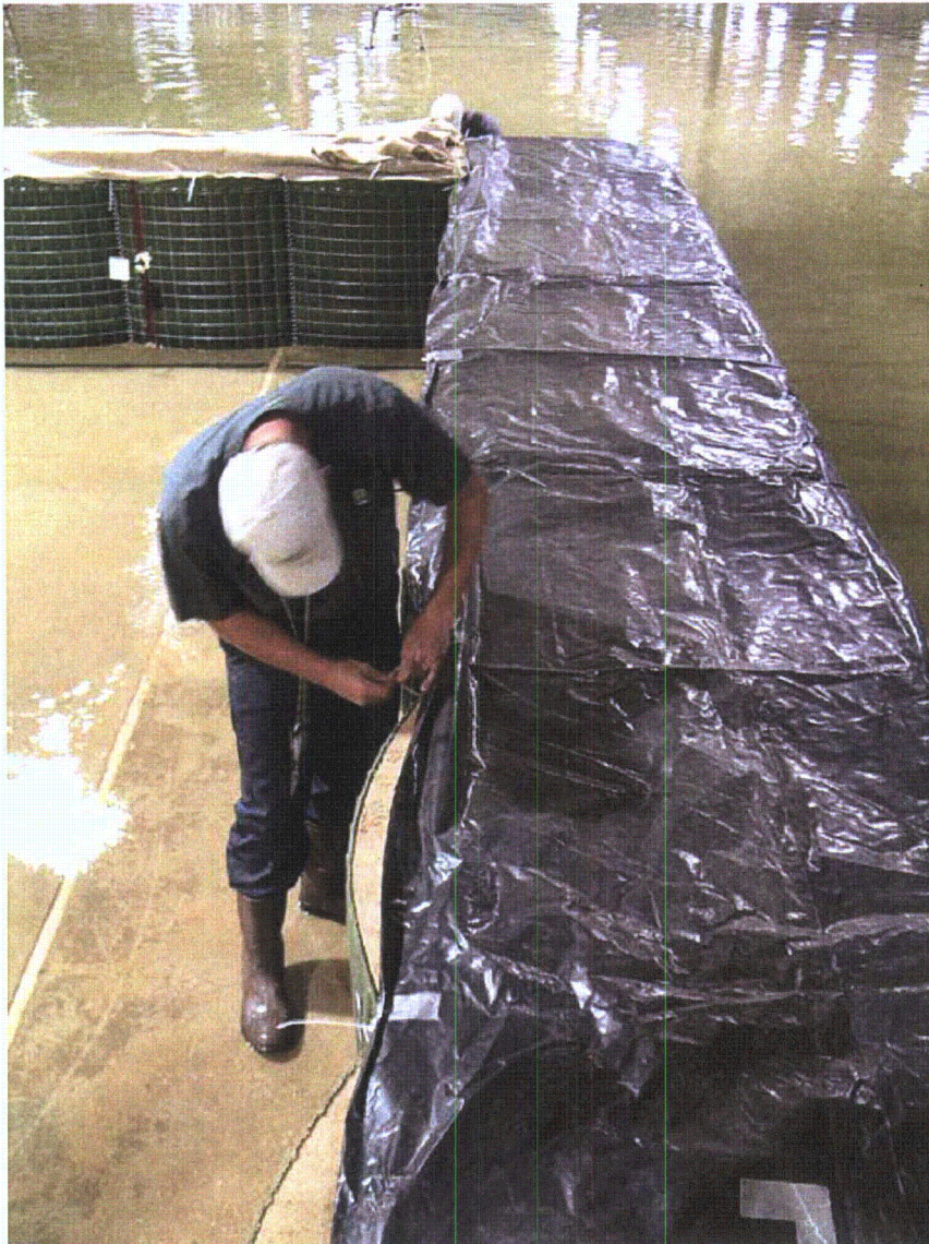
Figure 2-87. Repair 1, view along right wall
