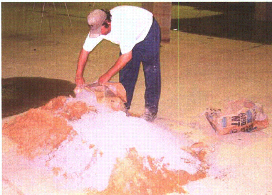
Figure 2-115. Mixing cement and sand for placement in toe grid cells
