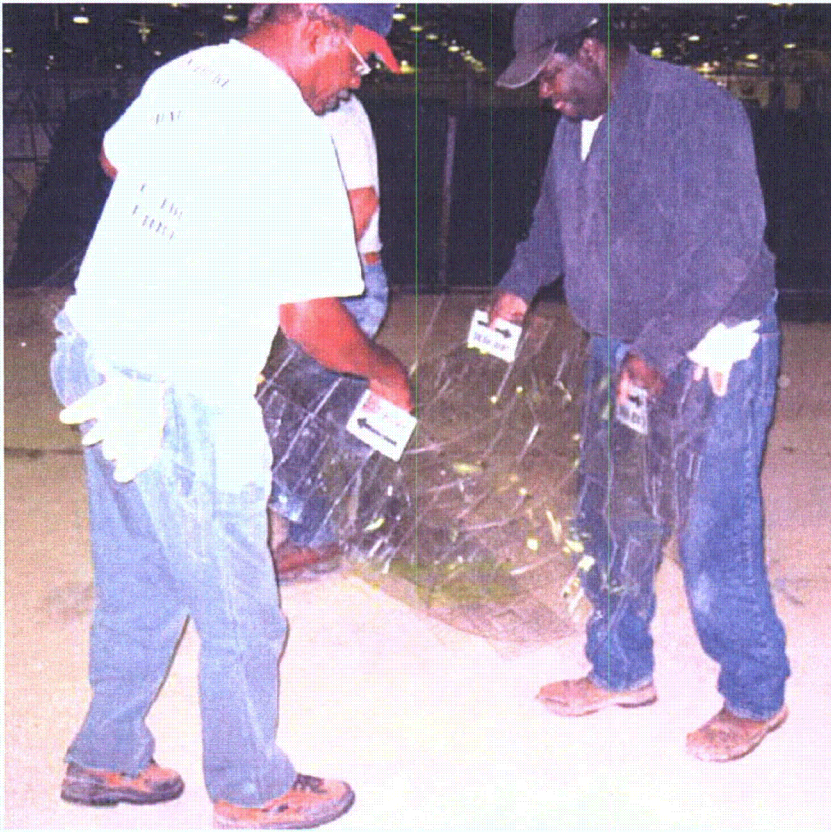
Figure 2-101. Removing and preparing to expand a grid unit
