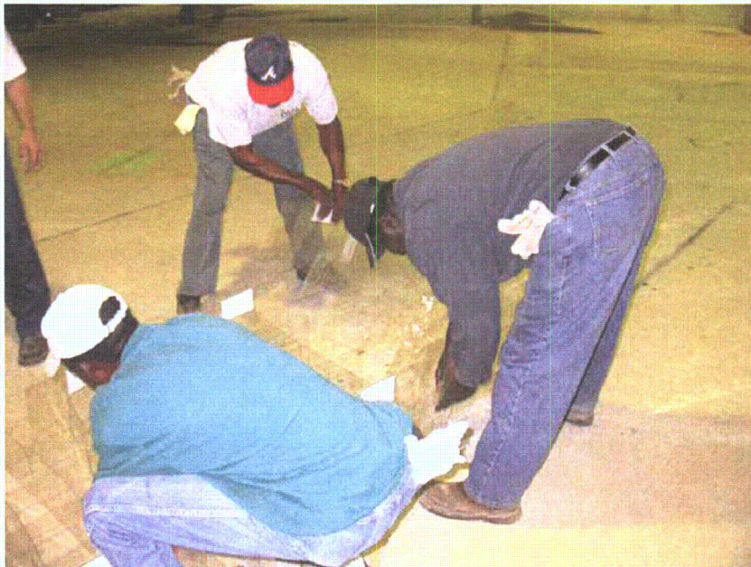
Figure 2-102. Laying expanded grid unit on floor
