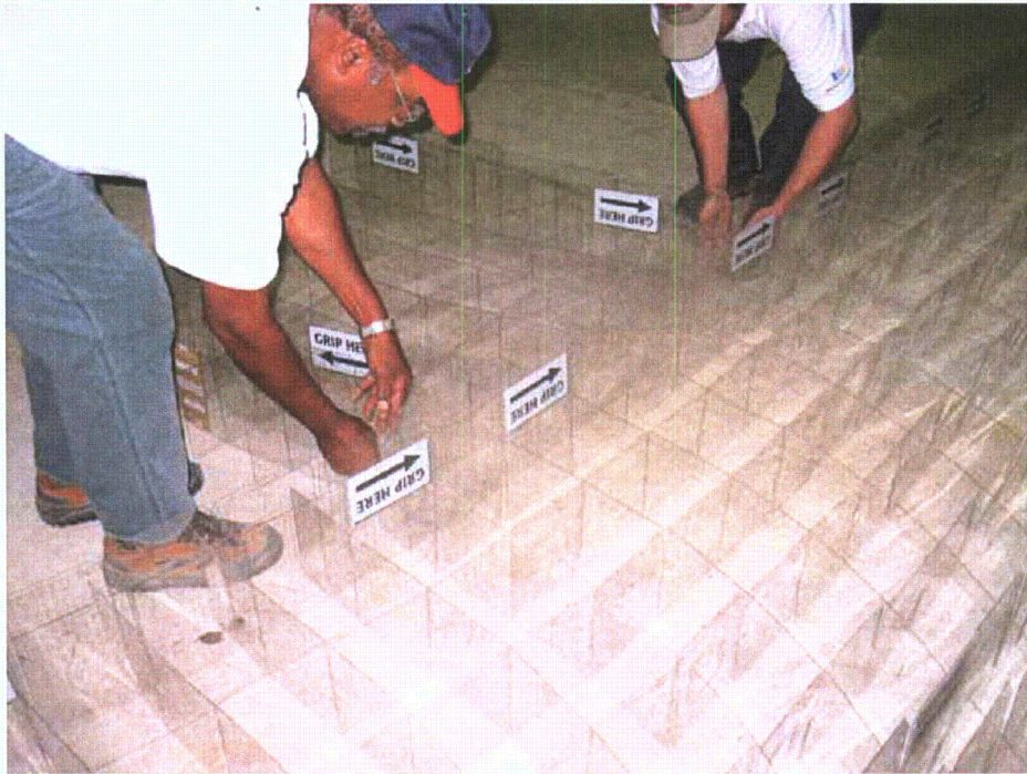
Figure 2-107. Connecting right wall to center wall grid cells, viewed from pool side
