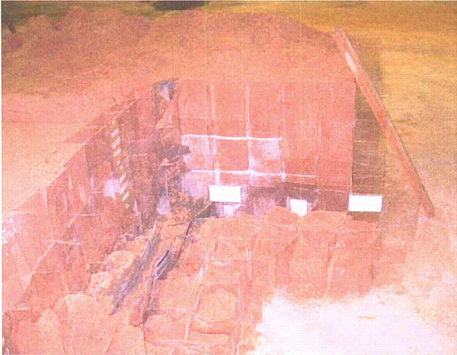
Figure 2-122. Right wall buttress viewed from pool side
