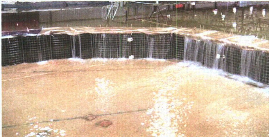
Figure 2-83. Overtopped levee structure, view from right wall
