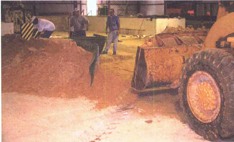
Figure 2-95. Removing sand pile
