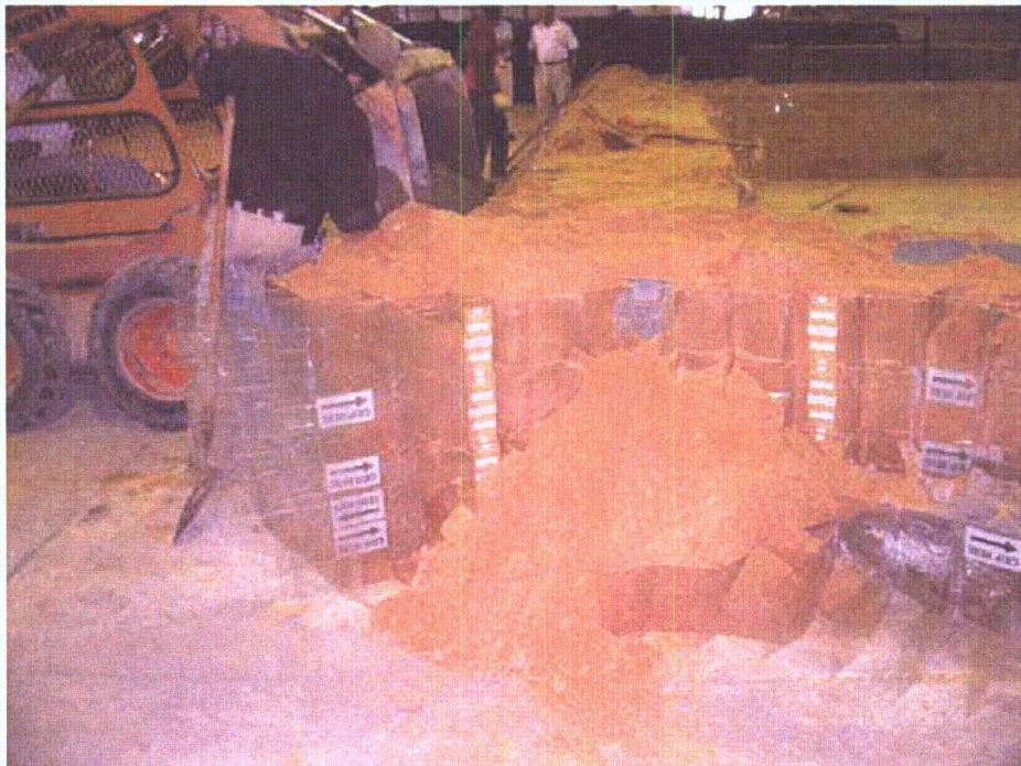
Figure 2-119. View of left wall/center wall buttress from pool side
