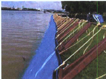
Figure 3-162. 8 June 2004, 2.7 ft of water against structure
