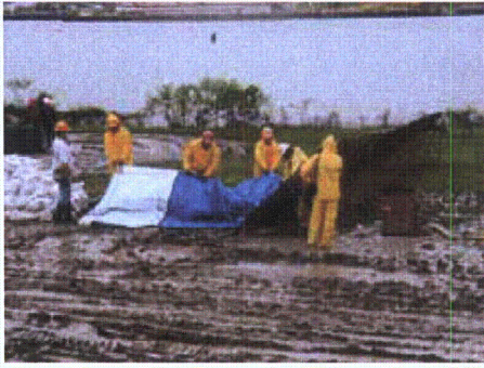
Figure 3-149. Unrolling liner membrane
