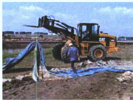
Figure 3-185. Forklift removing liner from excavated trench
