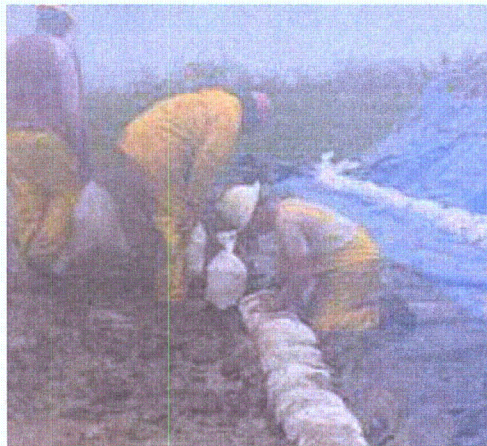
Figure 3-155. Placing sandbags on liner leading edge
