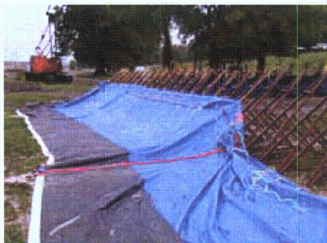
Figure 3-151. Liner membrane tied to support frame
