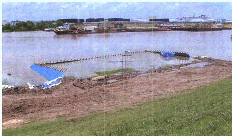
Figure 3-176. Portadam structure after protected side filled with water
