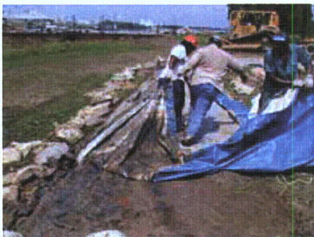
Figure 3-184. Laborers removing liner from excavated trench
