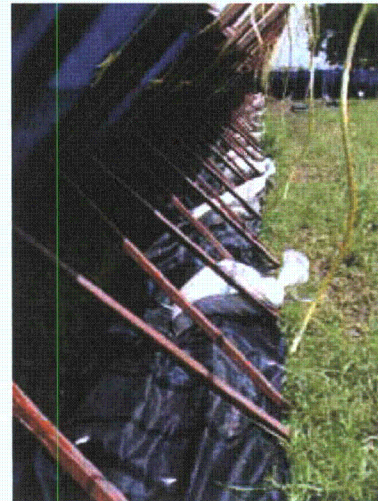
Figure 3-170. Typical preparation for overtopping (plastic sheeting)
