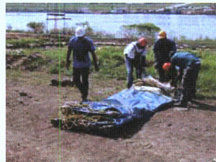
Figure 3-187. Rolling folded liner
