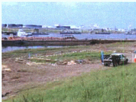
Figure 3-190. Portadam site with only sandbags remaining
