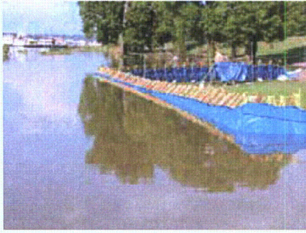
Figure 3-164. 10 June 2004, 3.5 ft of water against structure
