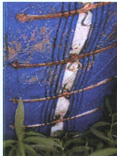
Figure 3-173. Stressed liner seam
