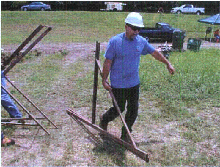
Figure 3-181. Carrying frame members to staging area
