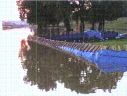
Figure 3-165. 11 June 2004, structure overtopped
