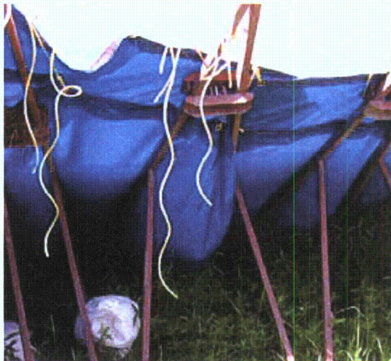
Figure 3-172. Sagging of liner between supporting frame members
