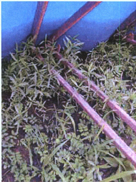
a. Unsunk frame along east tieback
