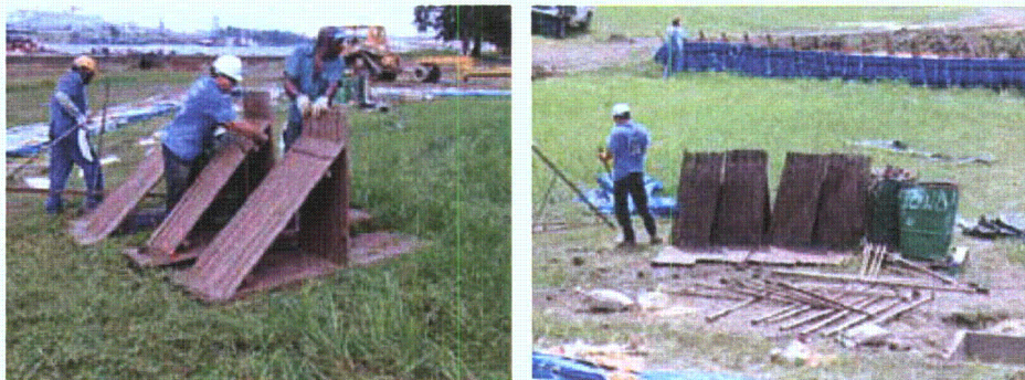
Figure 3-182. Removal staging area
