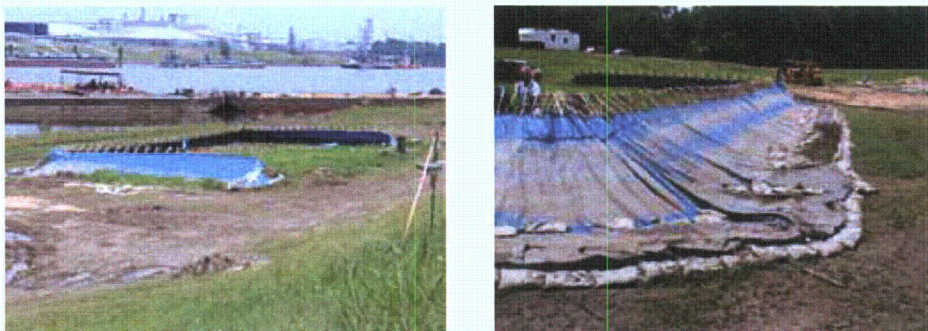
Figure 3-177. Portadam structure prior to removal
