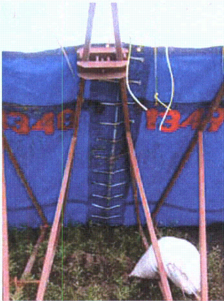
Figure 3-150. Seam between liner membrane sections
