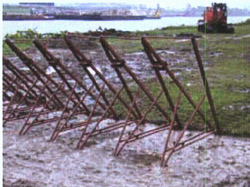
Figure 3-146. Supporting frame with bolts, clamps, and link bars (hardware)
