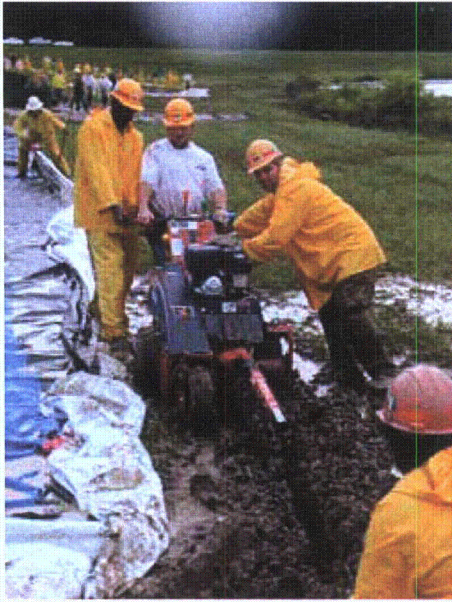
Figure 3-152. Excavating trench for liner leading edge
