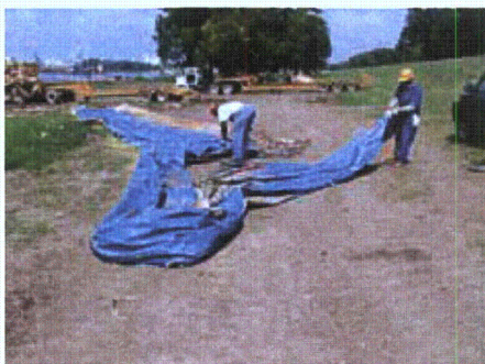
Figure 3-186. Folding liner
