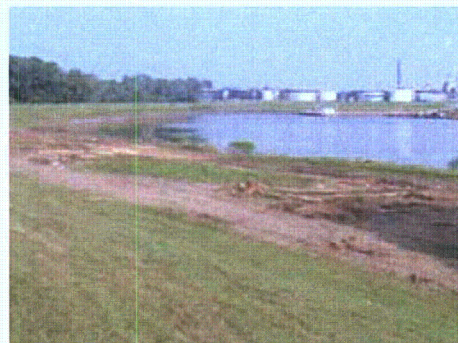
Figure 3-191. Portadam site after removal complete
