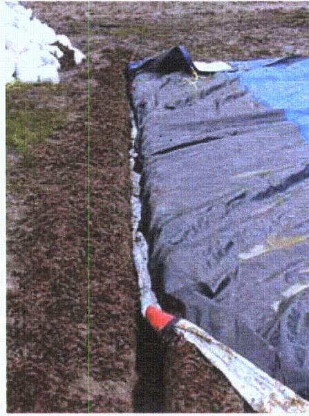
Figure 3-153. Liner leading edge placed in trench
