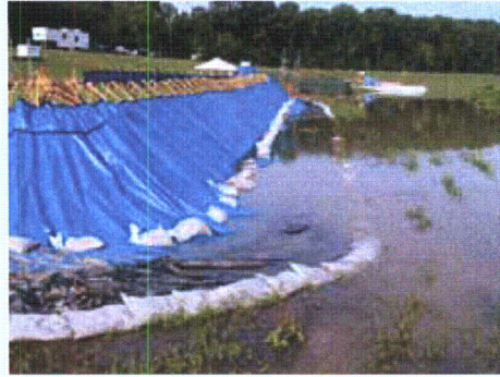
Figure 3-159. 5 June 2004, 0.3 ft of water against structure
