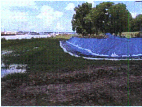
Figure 3-158. 4 June 2004, no water against structure
