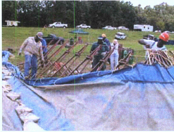
Figure 3-178. Removing liner membrane from supporting frame
