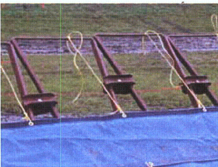
Figure 3-150. Seam between liner membrane sections
