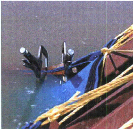
Figure 3-169. Sagging liner repair (repair 2)
