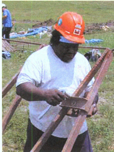
Figure 3-179. Disassembling supporting frame (bolts and clamps)
