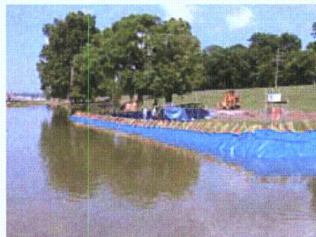
Figure 3-163. 9 June 2004, 3.1 ft of water against structure
