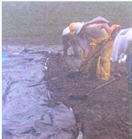
Figure 3-154. Burying liner leading edge
