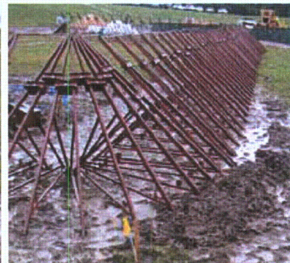
Figure 3-147. Structure frame constructed on graded and undisturbed ground
