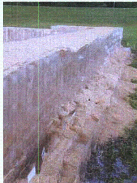
Figure 3-116. Riverward face of completed structure
