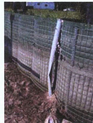
f. Bentonite-filled pipes after water receded
