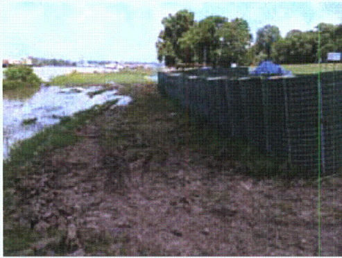
Figure 3-80. 4 June 2004, no water against structure
