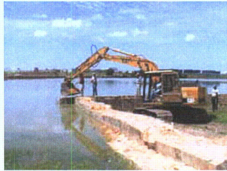
Figure 3-125. Trackhoe replacing sand field
