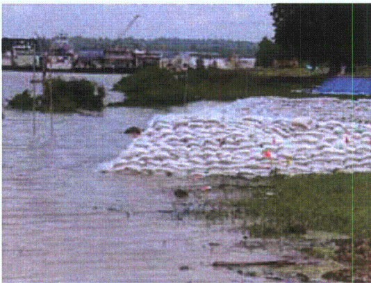
Figure 3-45. 4 June 2004, 1.0 ft of water against structure
