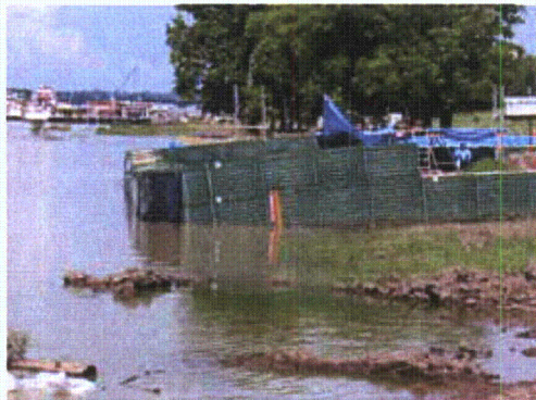
Figure 3-84. 8 June 2004, 2.7 ft of water against structure
