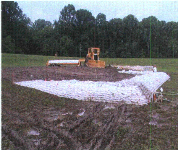
Figure 3-42. Completed 3-ft structure
