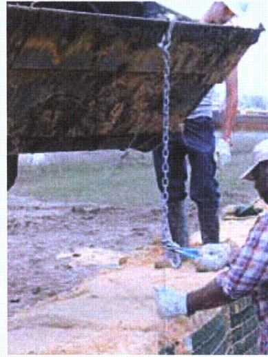
Figure 3-101. Removal of joint-connection pins with front-end loader
