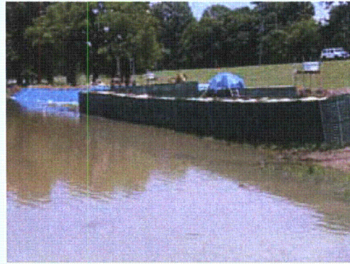
Figure 3-81. 5 June 2004, 0.3 ft of water against structure
