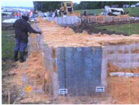
Figure 3-113. Filling of riverward face and east tieback section units
