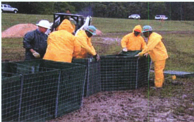
Figure 3-70. Installation of base row units
