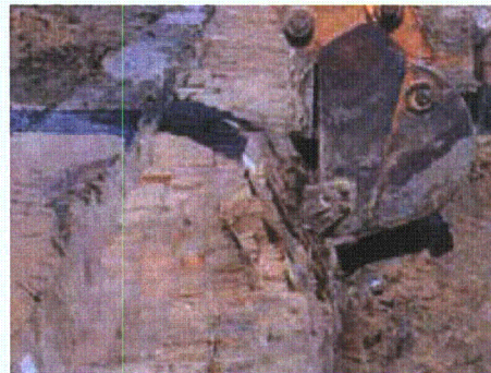
Figure 3-142. Removal with backhoe
