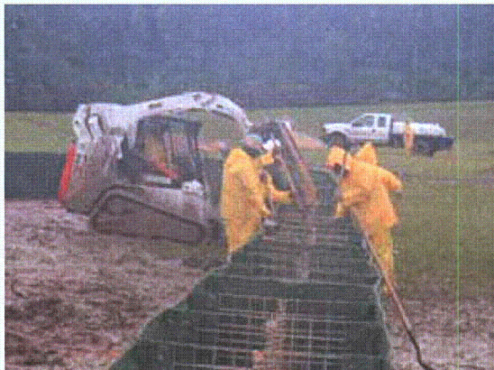
Figure 3-74. Filling base row with sand
