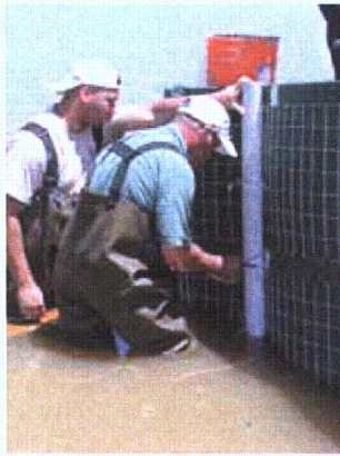
a. Attaching pipe to joints
