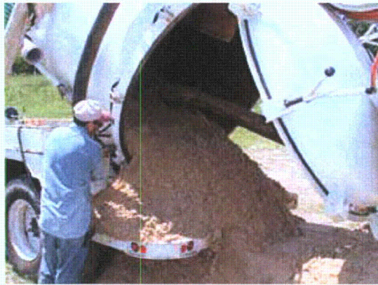
Figure 3-140. Removal of sand from truck
