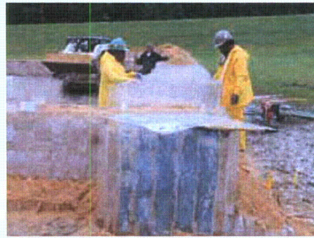
Figure 3-114. Installation of top row units (required raise)
