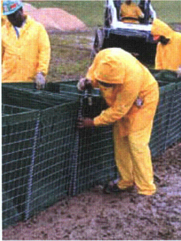
Figure 3-72. Installation of joint pins
