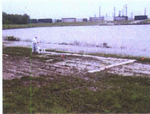
Figure 3-35. Laying first row of bags
