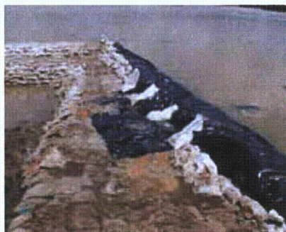
a. Prior to overtopping
