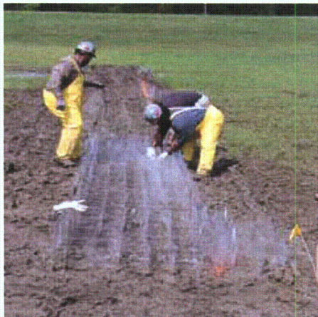
Figure 3-108b. Installation of RDFW base row
