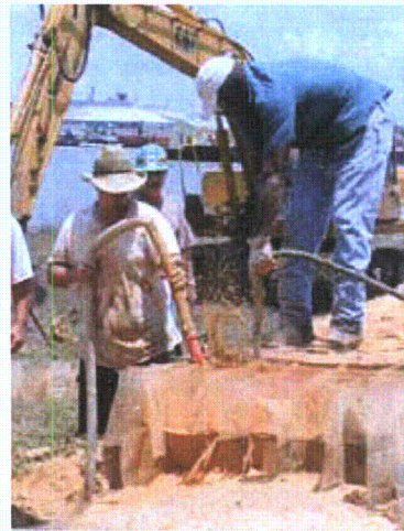
Figure 3-134. Sand removal from RDFW structure with water hose and compressed air
