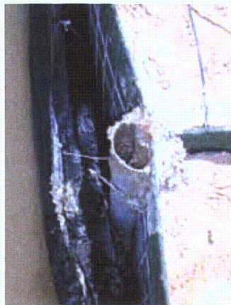
d. Pipe with bentonite
