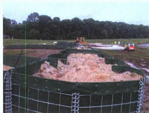
Figure 3-77. Sand fill in top row units
