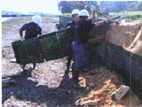
Figure 3-95. Removal of top row half units
