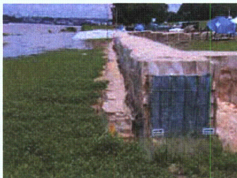
Figure 3-118. River level the day before testing began, 4 June 2004
