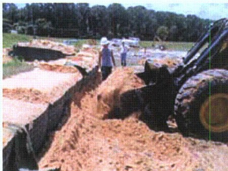
Figure 3-98. Removal of sand from around base row units
