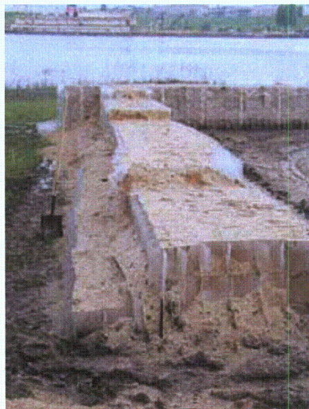
Figure 3-115. Sand fill in completed structure
