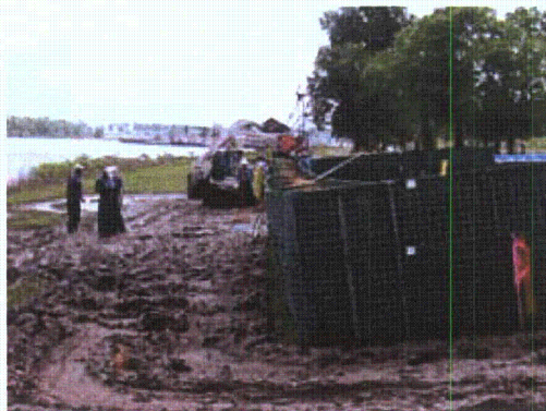
Figure 3-76. Filling top row units with sand
