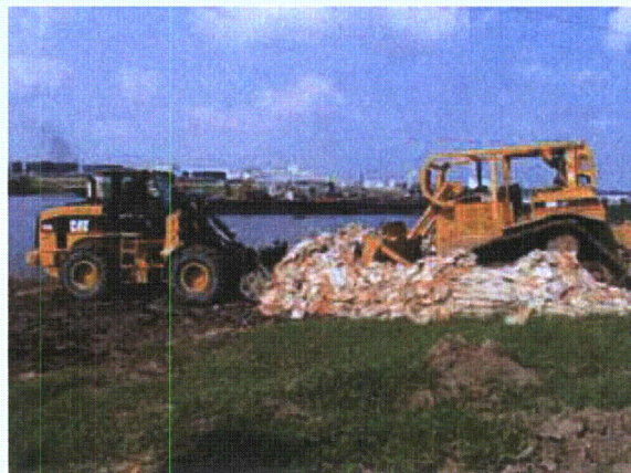
Figure 3-64. Dozer and front-end loader
