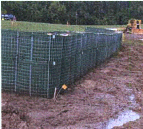
Figure 3-78. Riverward face of completed structure
