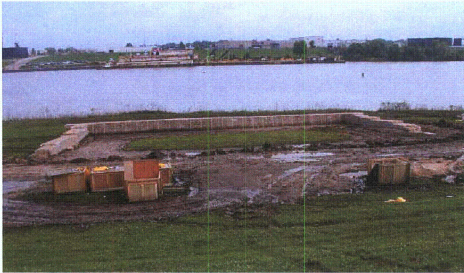
Figure 3-117. Completed RDFW structure
