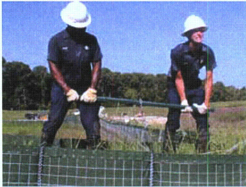
Figure 3-93. Removing center connection pins
