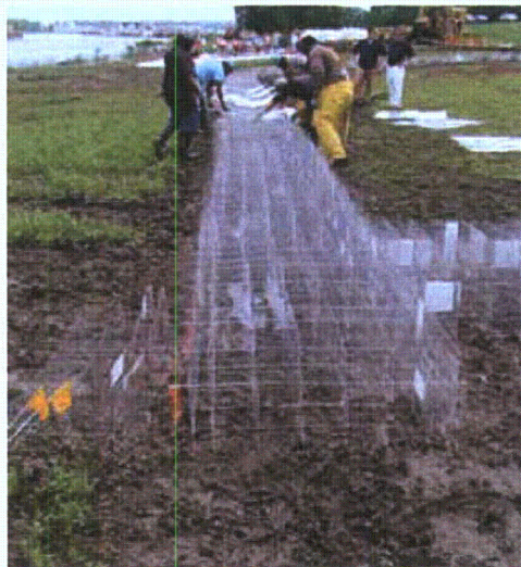
Figure 3-112. Filling of west tieback section units
