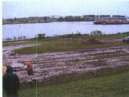
Figure 3-68. Hesco Bastion field site prior to construction
