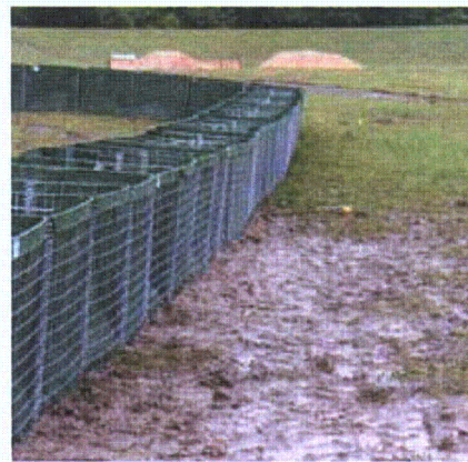
Figure 3-71. Structure constructed on graded ground and grass/weeds
