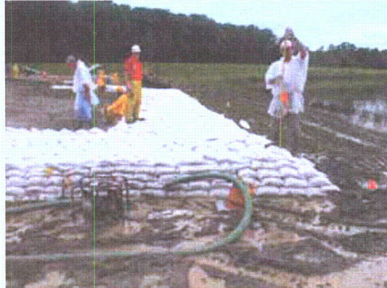
Figure 3-41. Measuring the height of structure
