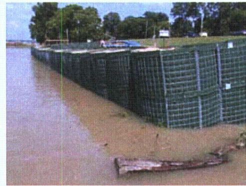
Figure 3-83. 7 June 2004, 2.1 ft of water against structure
