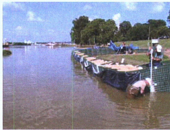
e. Packing bentonite into pipes
