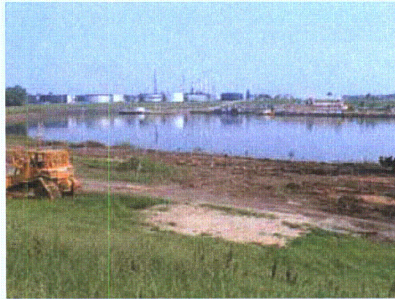
Figure 3-66. Structure completely removed
