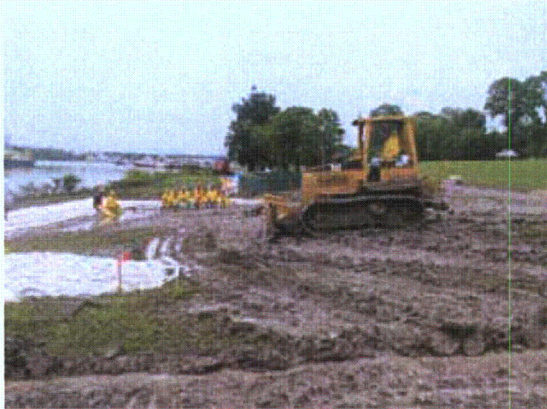
Figure 3-40. Area being backdragged to reduce mud
