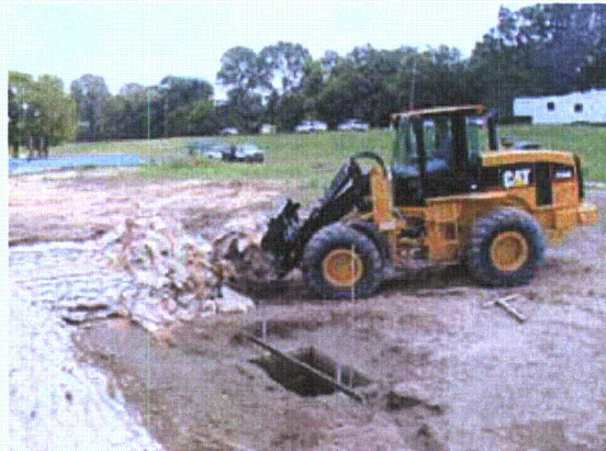
Figure 3-62. Sandbags removed by front-end loader
