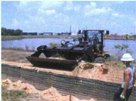
Figure 3-97. Removal of top row sand
