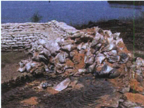
Figure 3-61. Removal of east tieback section
