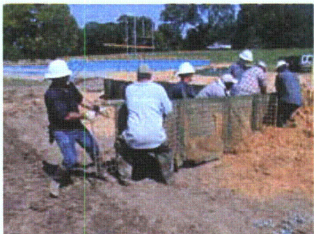
Figure 3-99. Removal of base row half units
