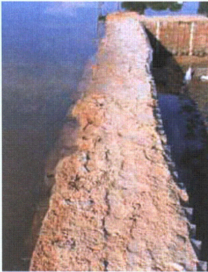
Figure 3-128. RDFW structure before overtopping
