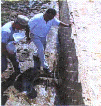
Figure 3-126. Using RDFW unit to contain sand boil
