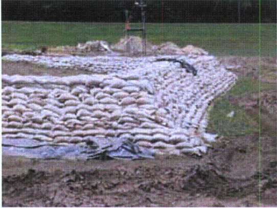
Figure 3-59. East side of structure
