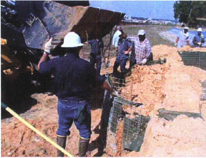
Figure 3-100. Removal of half units with front-end loader
