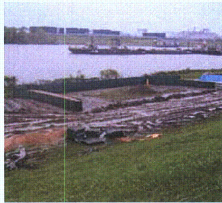
Figure 3-79. Completed structure from protected side
