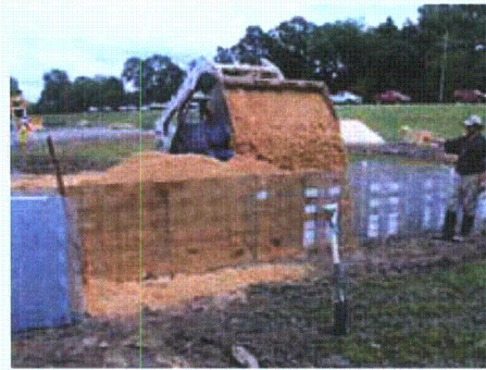
Figure 3-110. Installation of riverward face and tieback section
