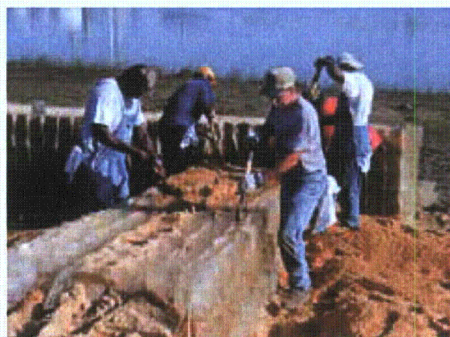
Figure 3-137. Removing sand with shovels
