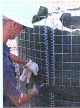
Figure 3-94. Removing zip ties
