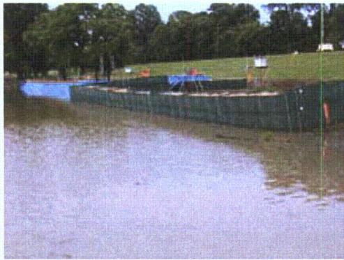
Figure 3-82. 6 June 2004, 1.3 ft of water against structure
