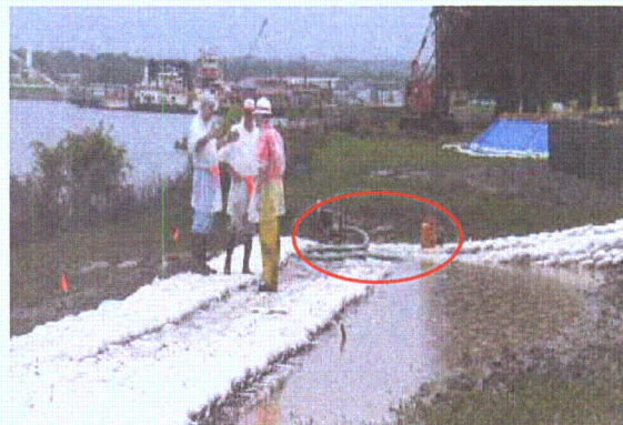
Figure 3-39. Water being pumped from structure
