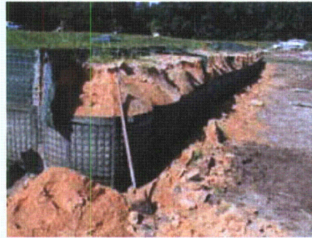
Figure 3-96. Riverward face of structure
