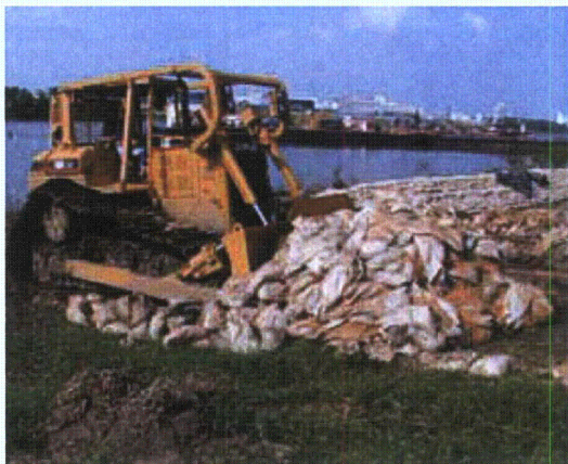
Figure 3-63. Bulldozer piling up sandbags
