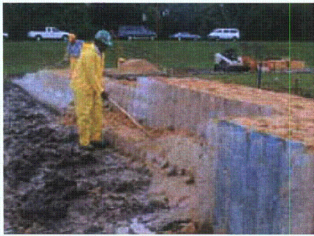
Figure 3-109. Installation of tieback section
