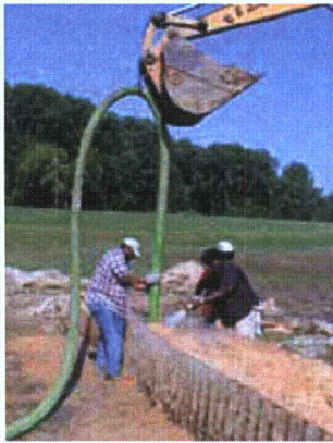
Figure 3-139. Vacuuming sand
