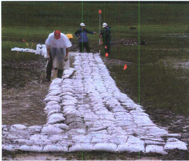
Figure 3-36. Partially completed riverward face, first row
