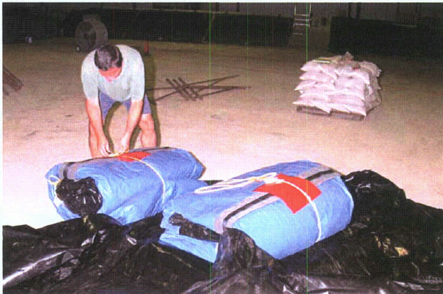
Figure 2-197. Offloaded vinyl tarp sections to begin unrolling operation
