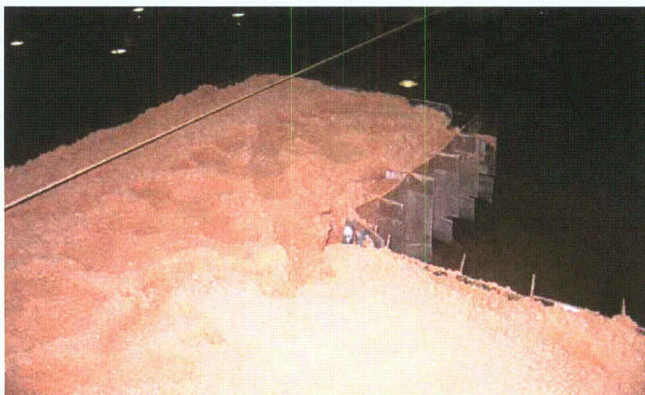
Figure 2-139. Right wall buttress
