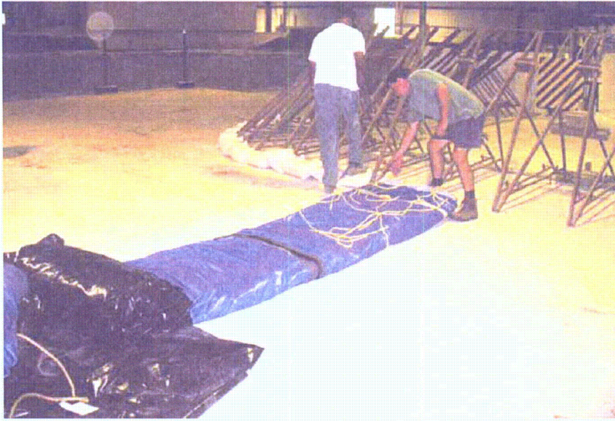
Figure 2-198. Unrolling tarp section
