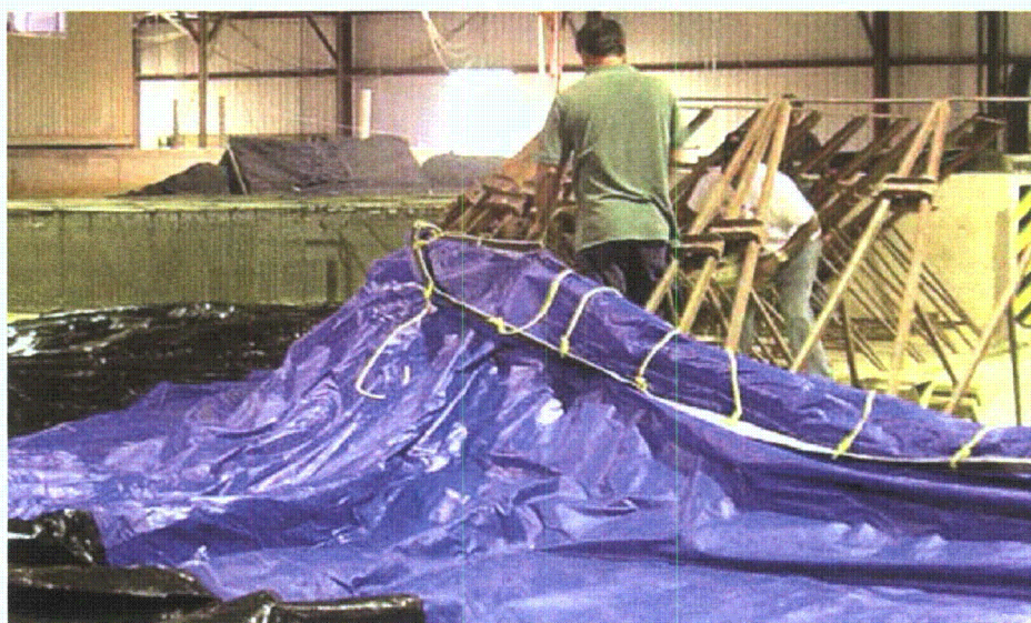
Figure 2-205. Pulling vinyl tarp up to frame
