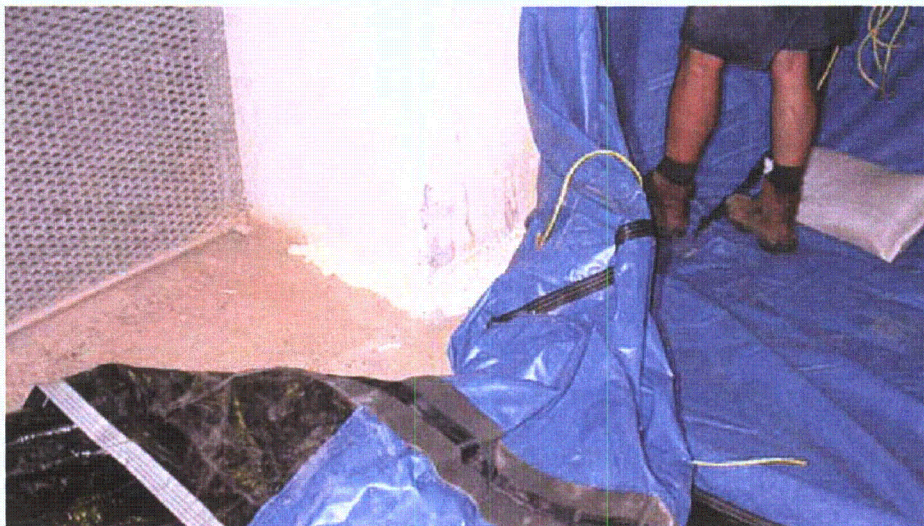
Figure 2-209. Expandable foam treatment at concrete wall abutment
