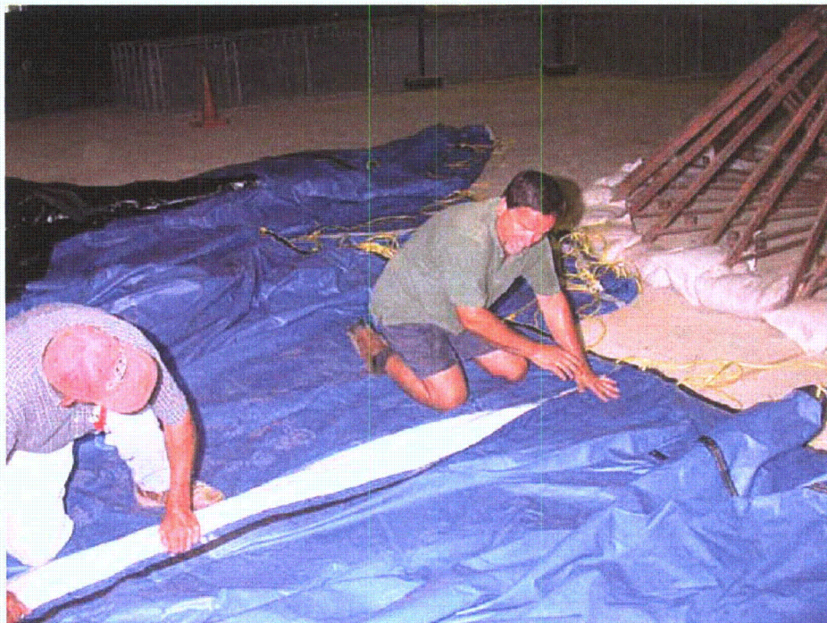
Figure 2-203. Hook and loop fastening seam flap
