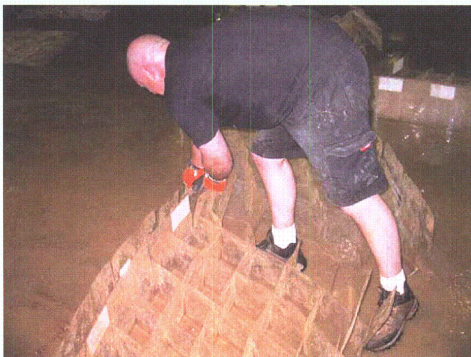
Figure 2-176. Disassembling grid unit for future reuse
