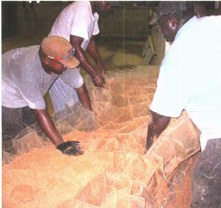
Figure 2-172. Pulling grid unit in an upward fashion
