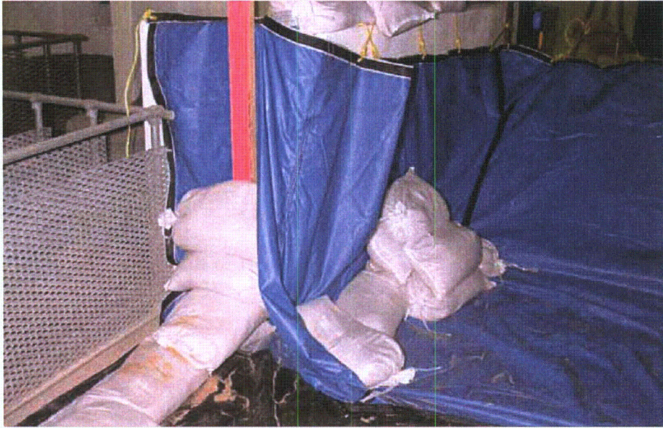
Figure 2-210. Sandbags and 2x4 board along concrete wall abutment
