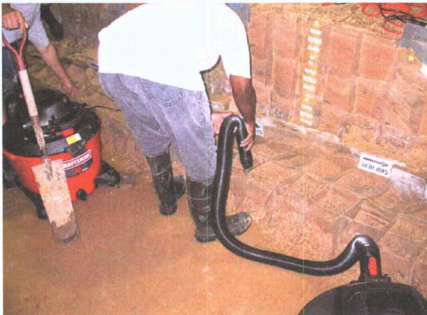
Figure 2-163. Vacuuming sand out of toe grid units
