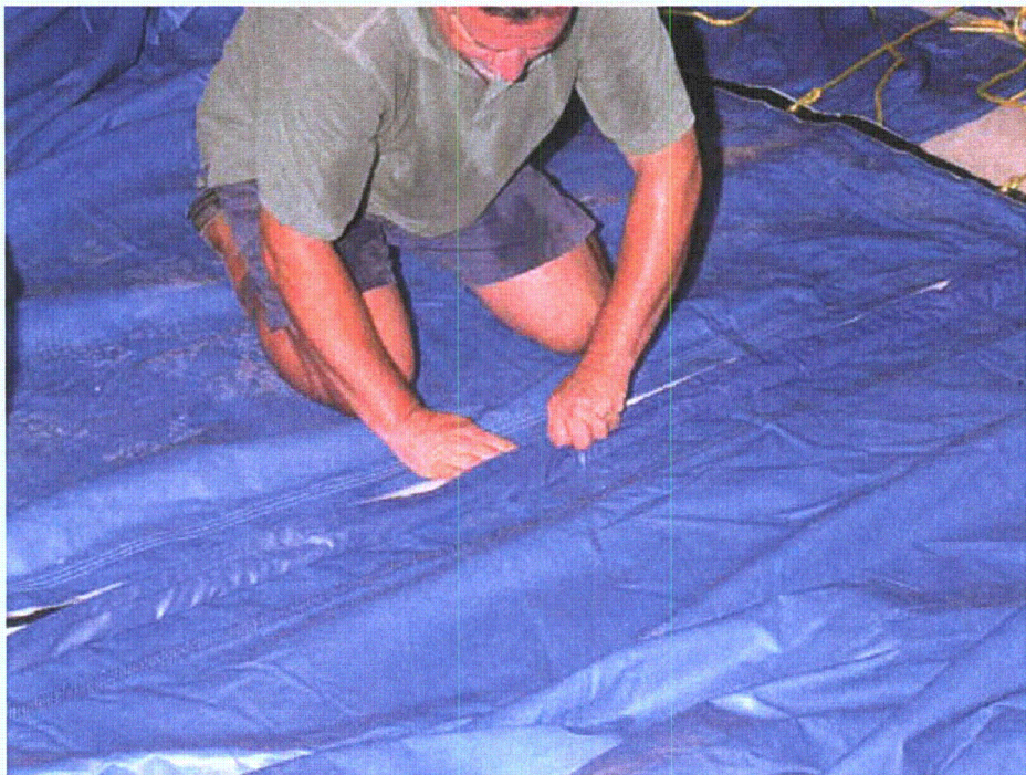
Figure 2-204. Vinyl tarp seam connection complete
