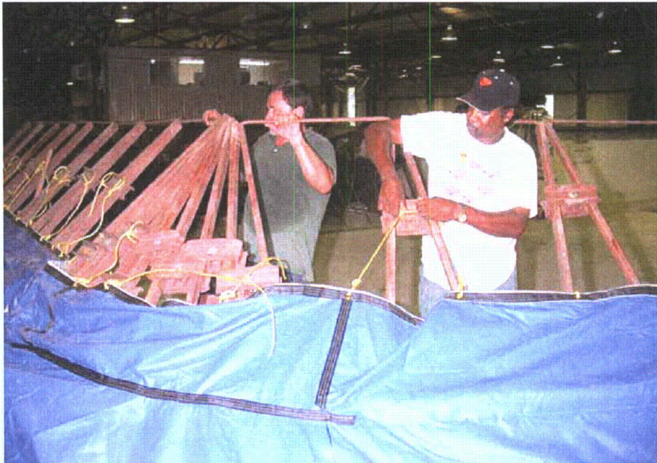
Figure 2-206. Tying tarp to frame
