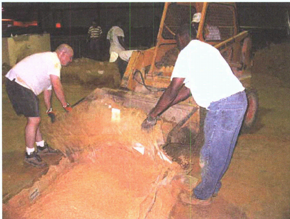
Figure 2-181. Bottom layer removal assistance provided by small loader
