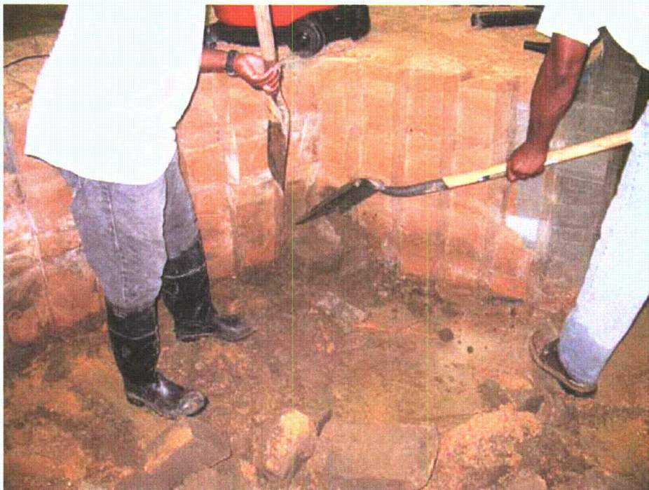
Figure 2-166. Cleaning out remaining toe grid materials
