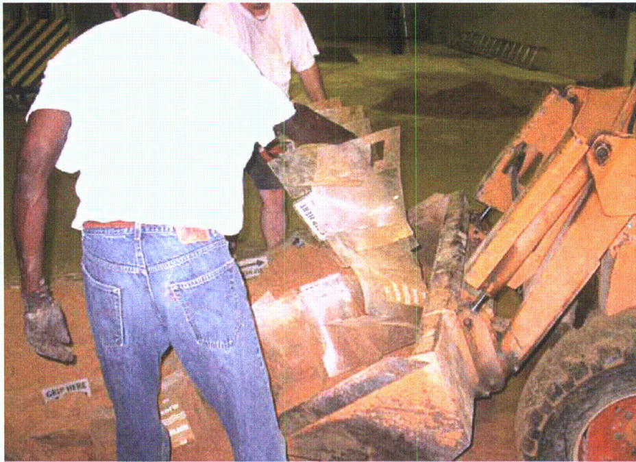
Figure 2-182. Removing grid unit/sand combination
