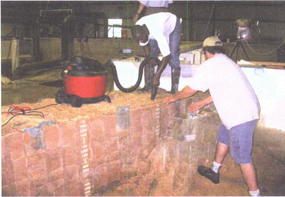
Figure 2-167. Removing sand from top of wall
