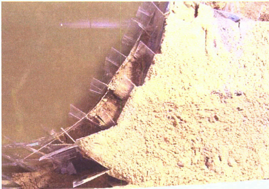
Figure 2-132. Left concrete wall abutment
