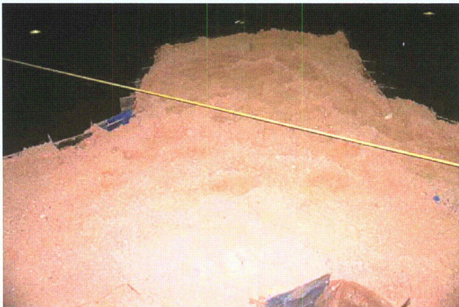
Figure 2-138. Left wall buttress
