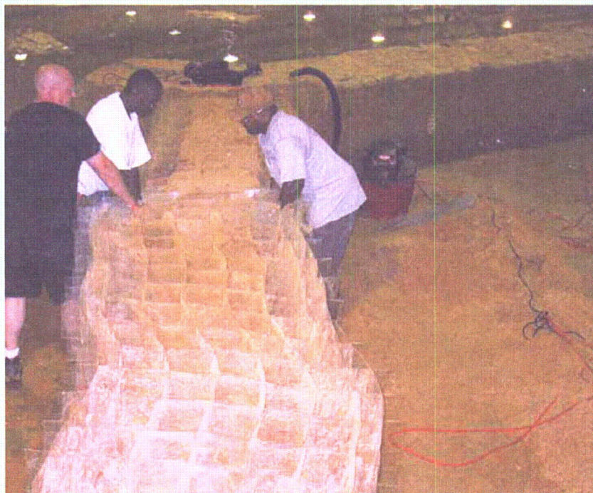
Figure 2-174. Loosening attached grid units
