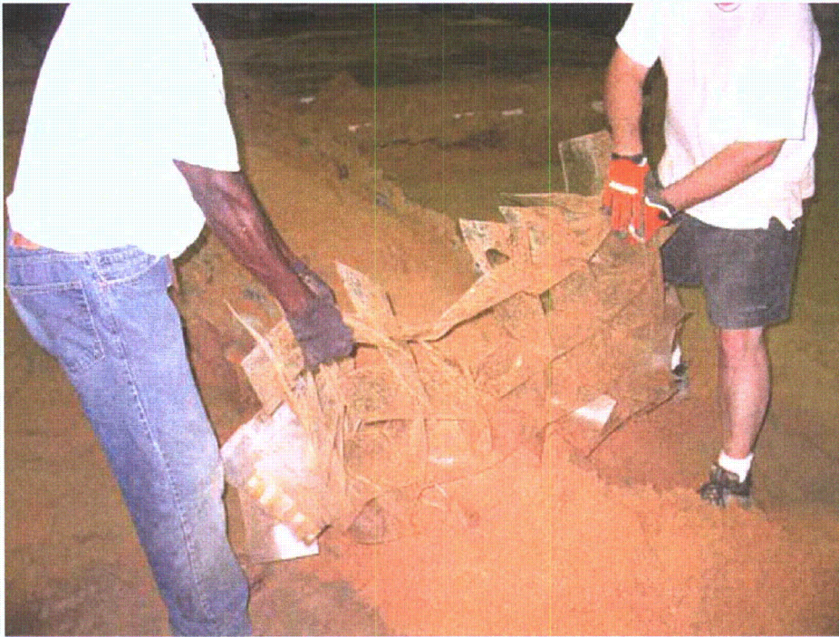
Figure 2-180. Removing a grid unit
