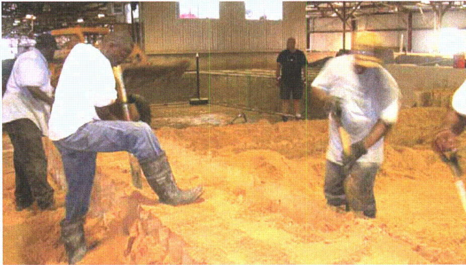
Figure 2-178. Continuation of sand removal using shovels
