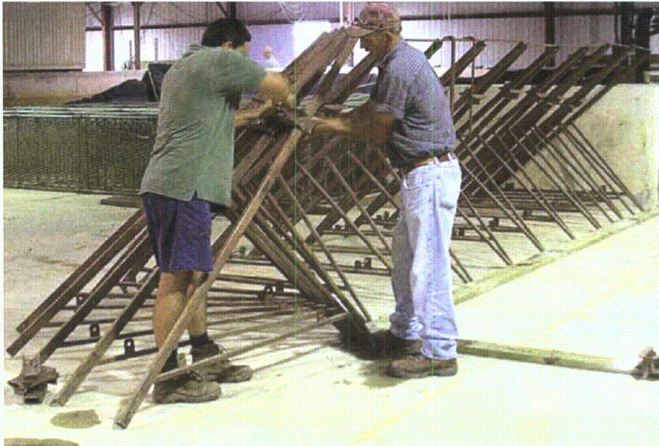
Figure 2-194. Installing frame at 90-deg corner
