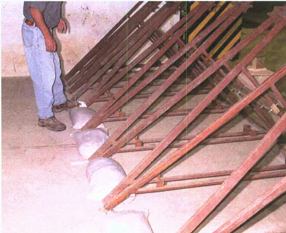
Figure 2-199. View of sandbags placed between each frame opening
