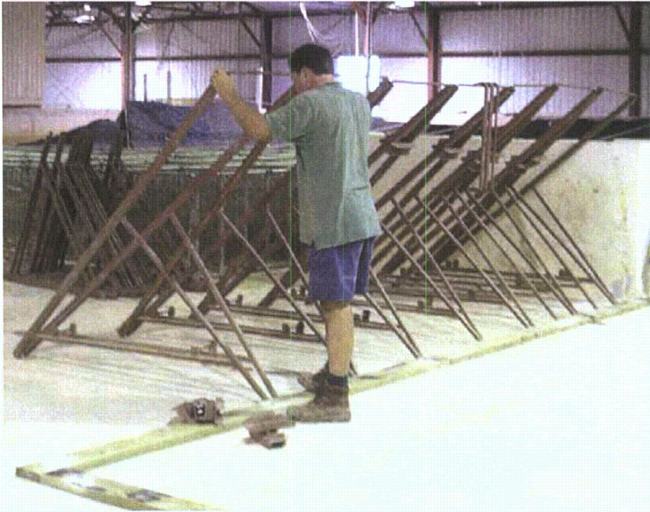
Figure 2-191. Beginning frame installation from right abutment wall
