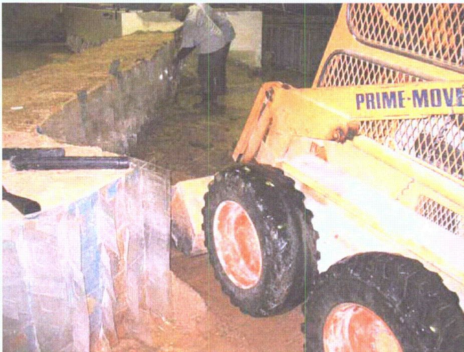
Figure 2-165. Removing toe grid materials
