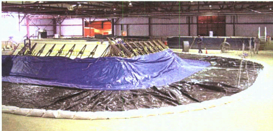
Figure 2-211. Portadam® levee construction completed
