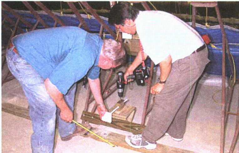
Figure 2-213. Installing one of laser targets
