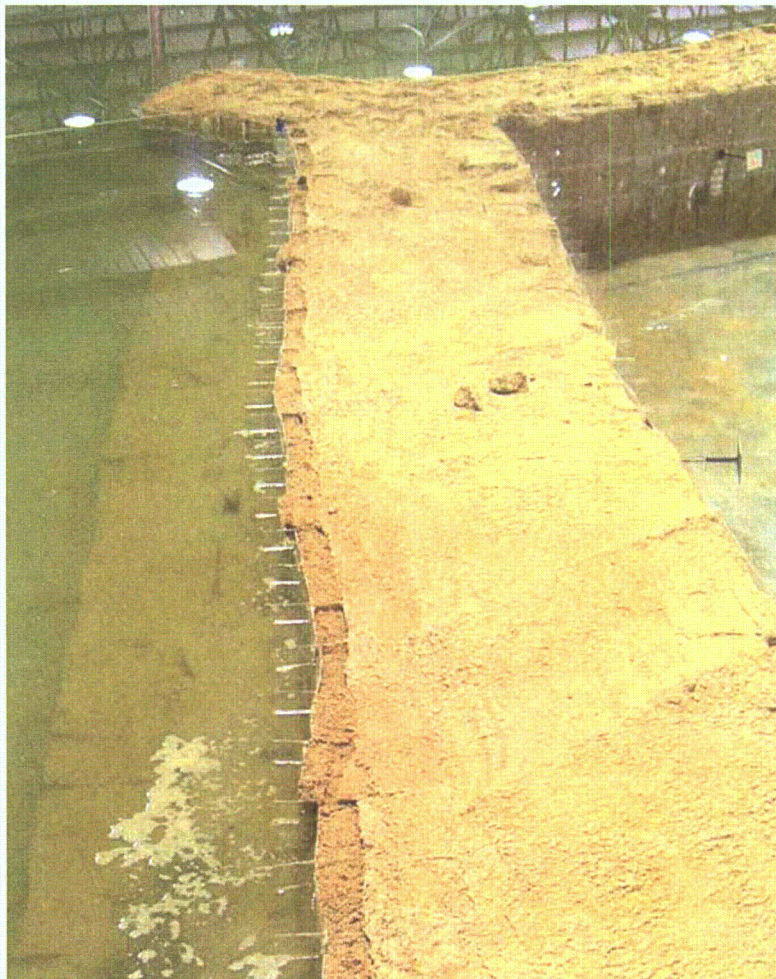
Figure 2-136. View looking down left wall
