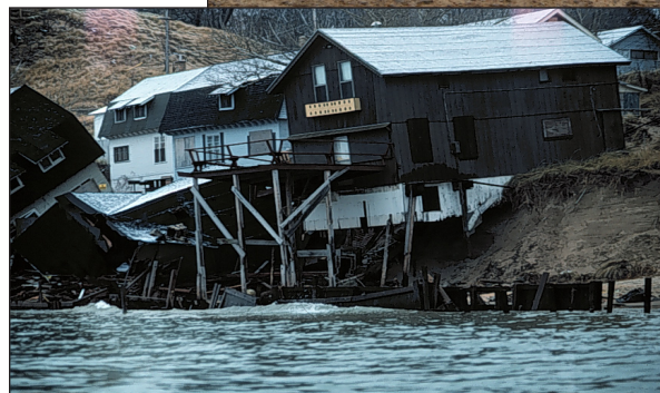
High lake levels on Lake Michigan in 1986 caused severe erosion.
