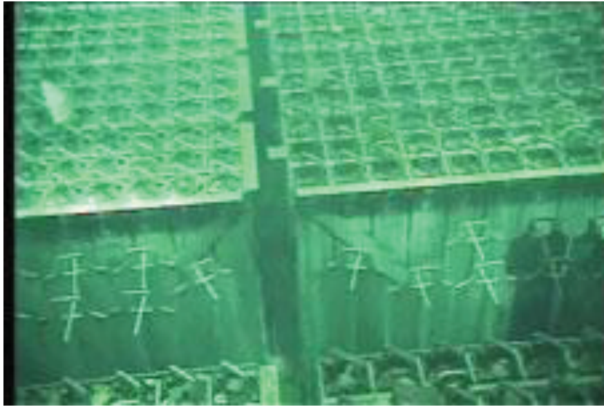
Fig. IV-5-12 Condition of the spent fuel pool (Unit 4)
