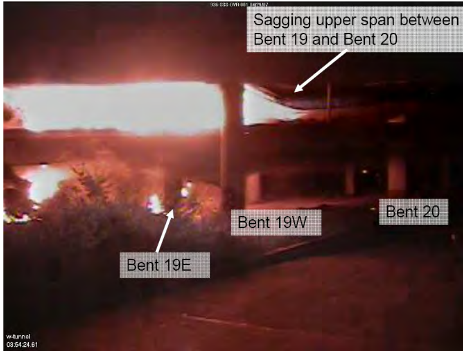
Figure 1. MacArthur Maze fire at +16.7 minutes (video image at 03:54:24.61 PDT)
