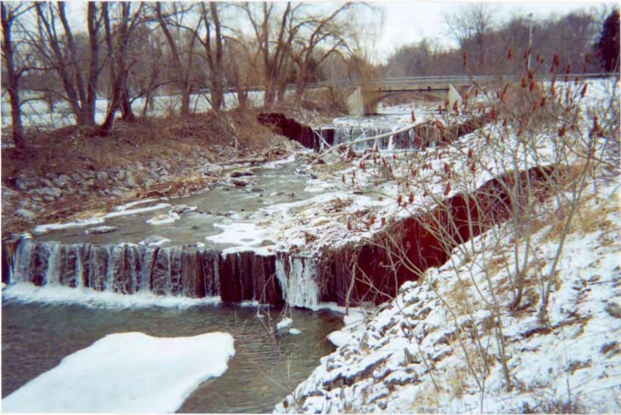
Figure 10. Sheet-pile Drop Structures
