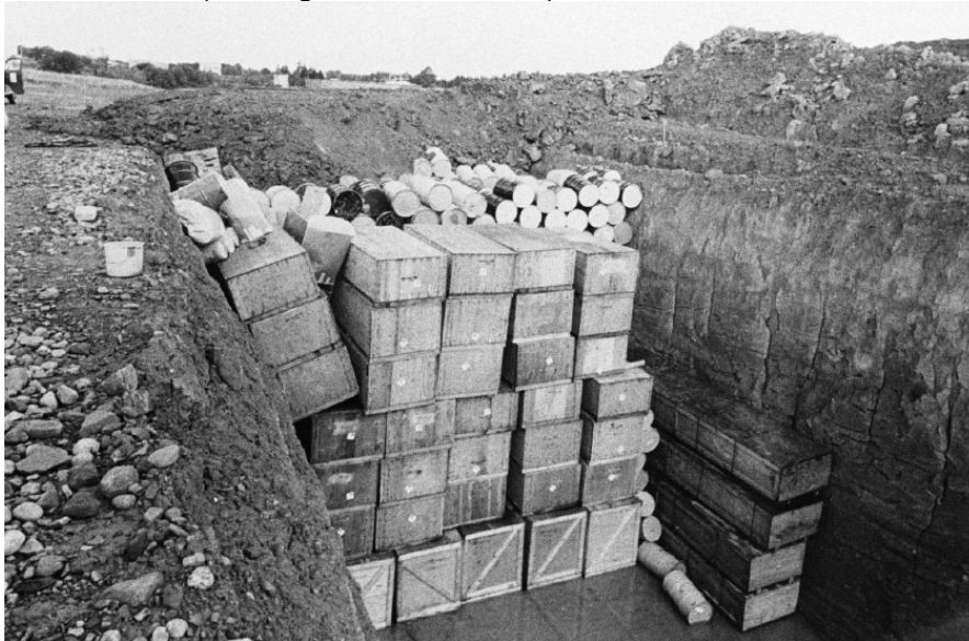
Figure 3.5 Photograph of wastes in wooden boxes and other canisters being loaded into a trench in State licensed Disposal Area (SDA).
