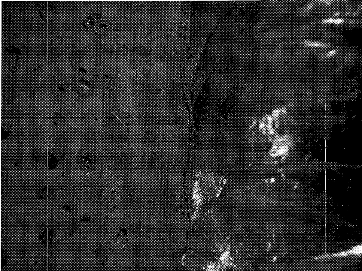
Figure 6 ID Surface Appearance of the Weld at the Carbon Steel Interface – Note the Presence of Pitting in the Carbon Steel at the Weld Heat Affected Zone and Cracking at the Weld Interface
