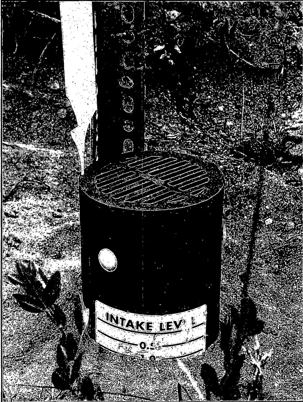
Figure 2.7-4. Stormwater sampler installed to collect a 1-L sample of snowmelt or storm surface runoff.
