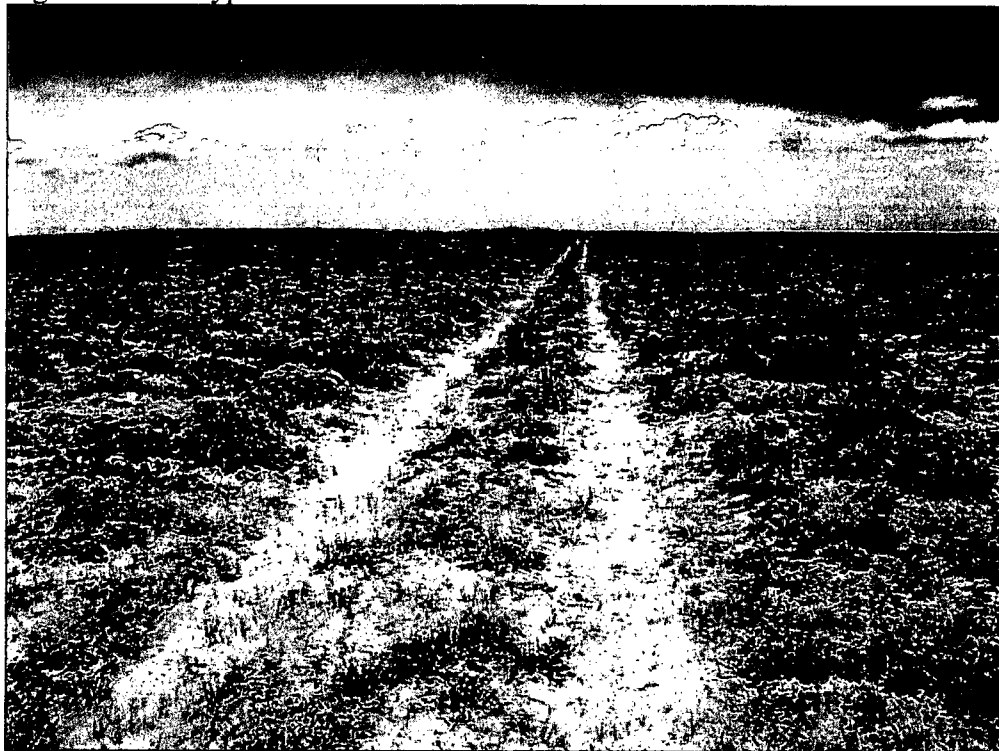
Figure 2.6-11 Typical Two-Track Road
