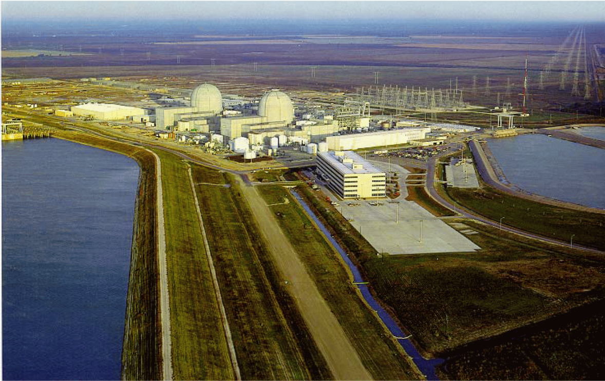
Figure 3.1-1 STP 1 & 2 with MCR on Left and Essential Cooling Pond on Right
