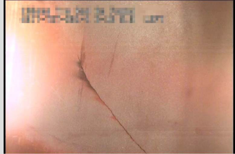
Discolorations at Crack Surface
