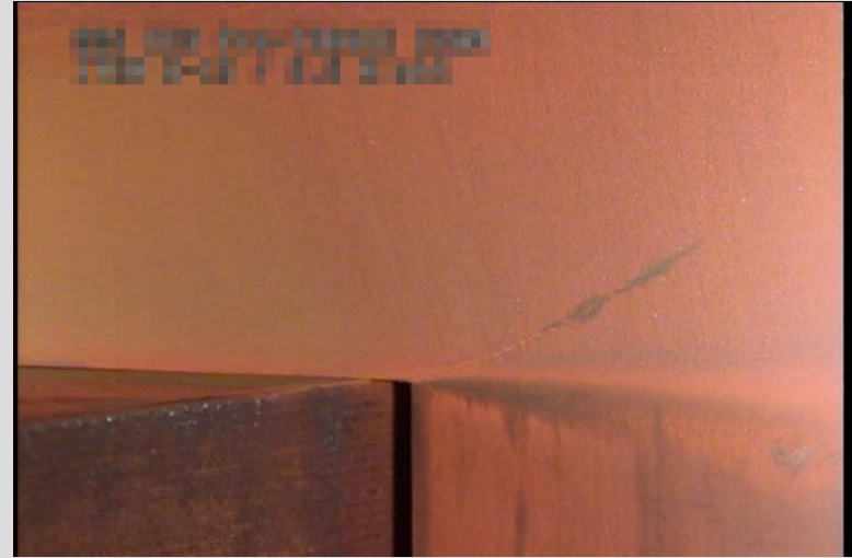
Possible Cracks
