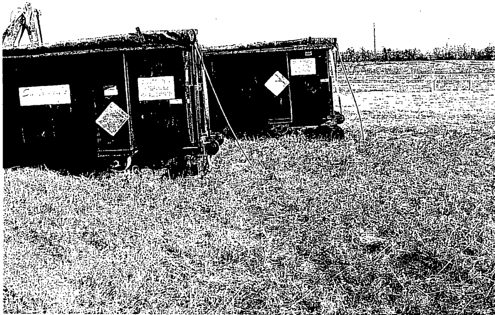
View of 20-yard roll off containers to be filled with contaminated soil
