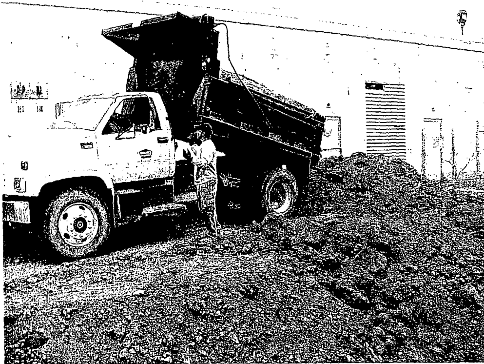
View of clean soil being hauled-in to the site
