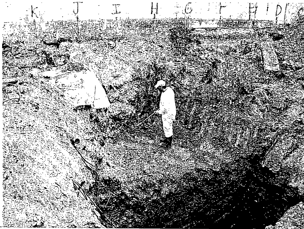
View of confirmation sampling in shallow portion of the excavation
