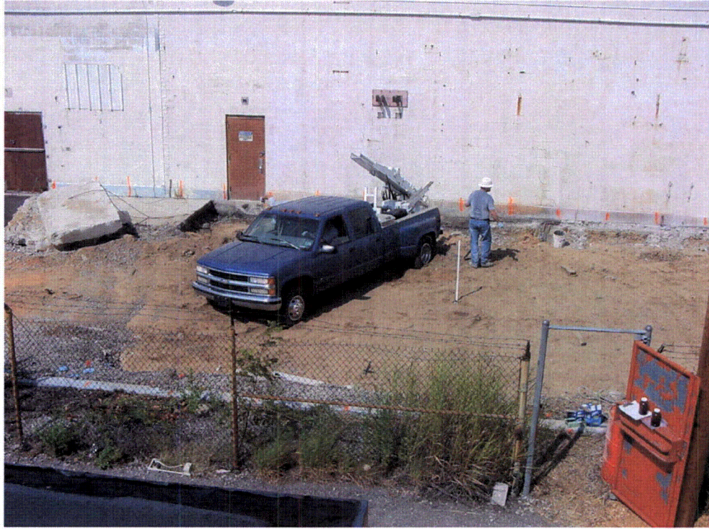
View of PCB Area during subsurface investigation
