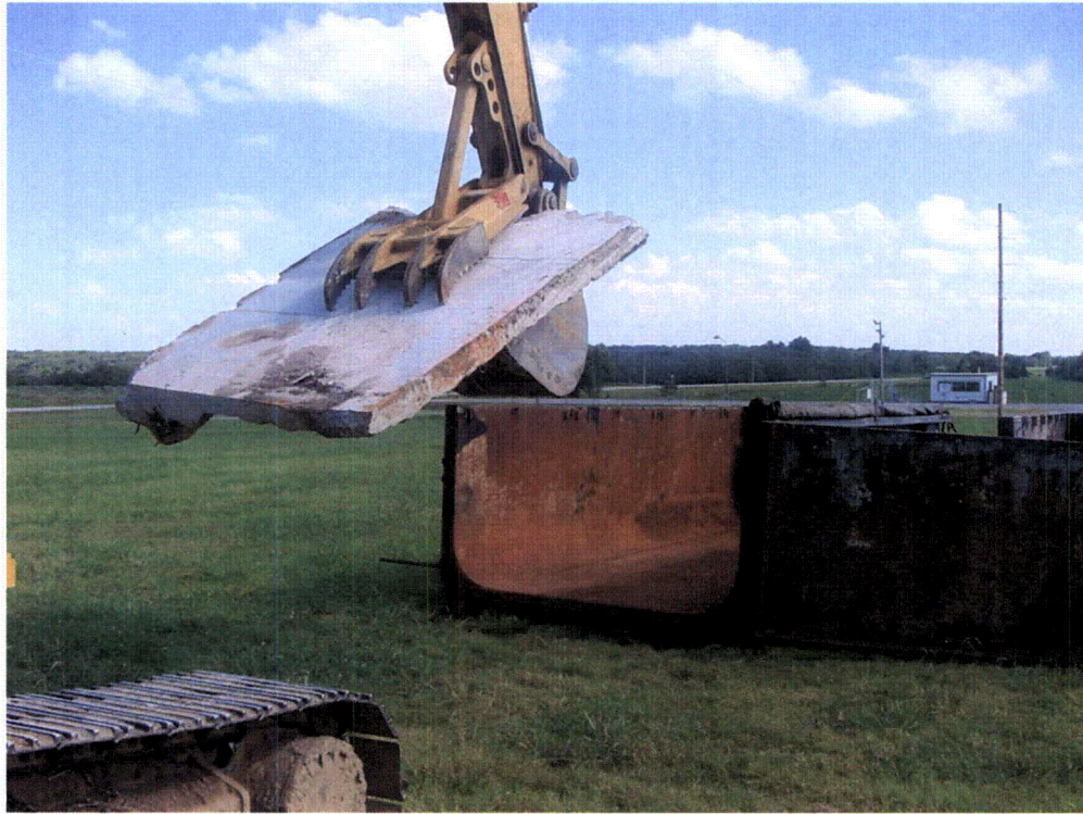
View of concrete slabs being loaded into roll-off containers
