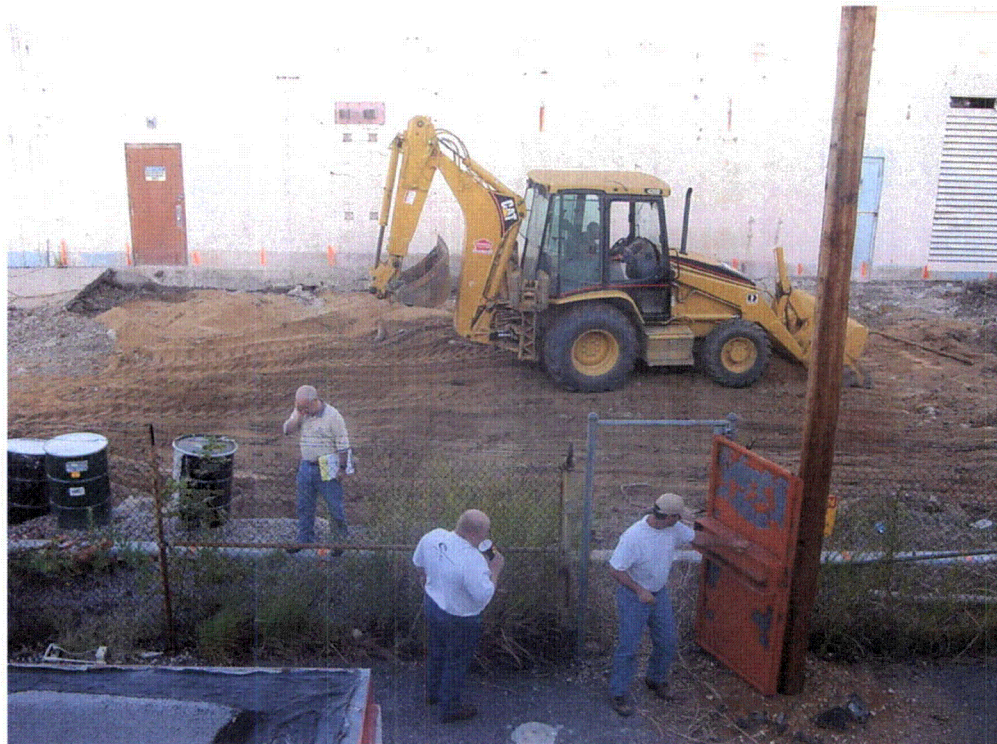
View of PCB Area after slab removal
