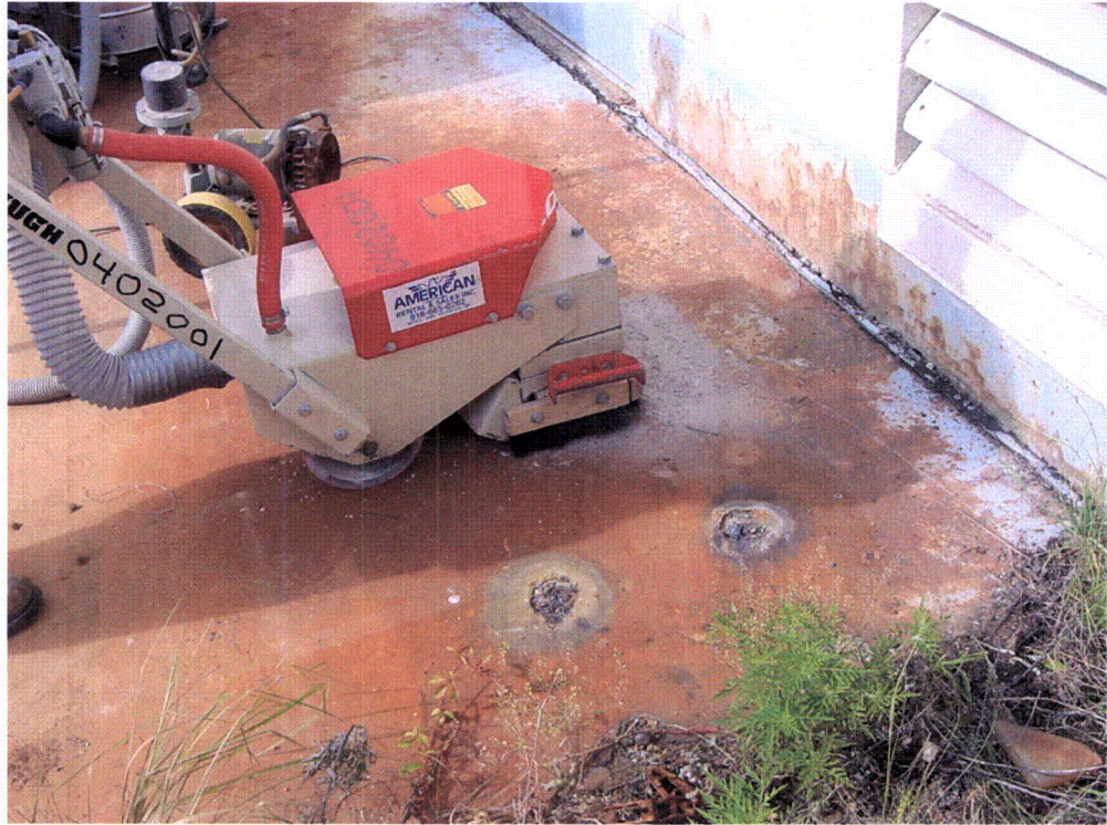
View of Scabblor removing concrete samples
