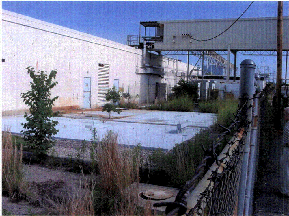
View of PCB Area with slabs looking northwest
