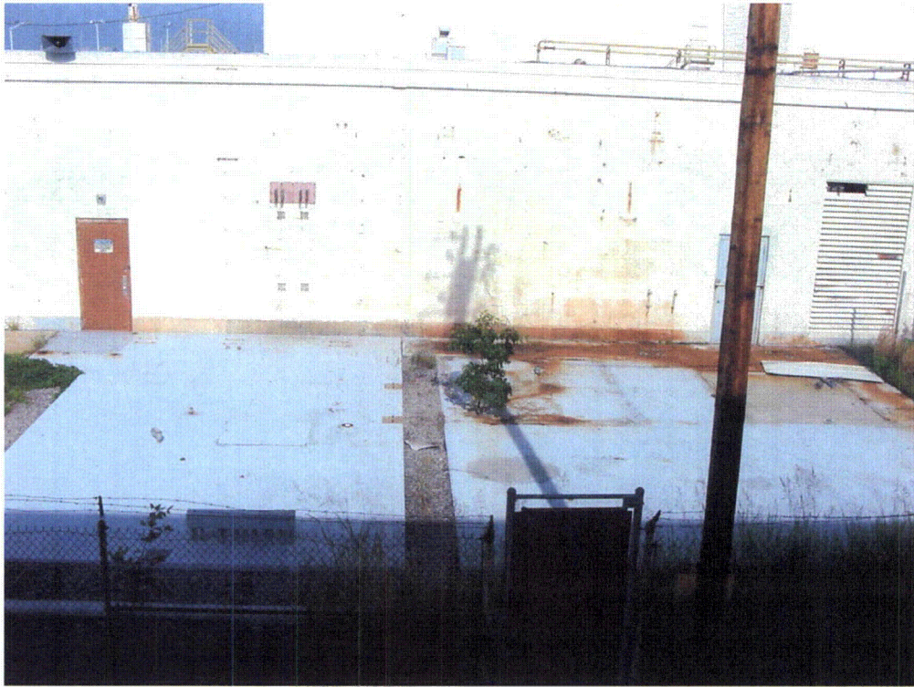
View of PCB Area with slabs looking west
