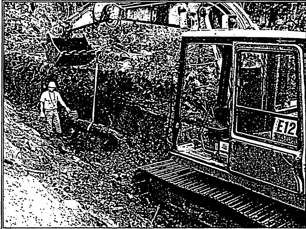
Removal of the SNEC WEIR Line Extension to the Raystown Branch of the Juniata River
