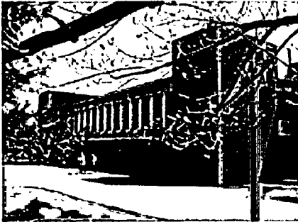
Science & Technology Building Niagara County Community College Sanborn, NY
