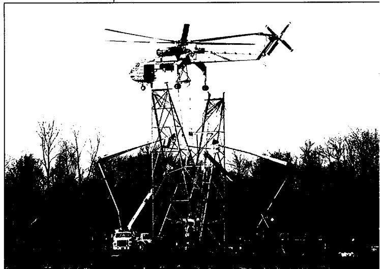
Serving the needs of 660,000 metro area St. Louis customers, a new transmission line extension went into service in 1999. At right, a helicopter delivers a section of a 326-foot steel tower for a 12.6-mile extension, linking AmerenUE's Sioux Plant in Missouri to an Illinois substation.
