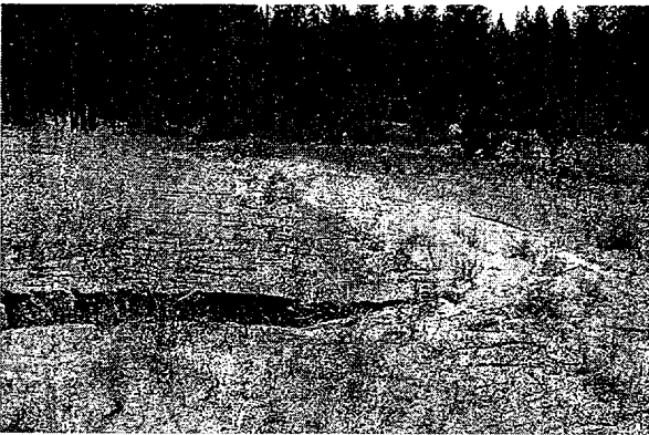
Photograph is of the south end of the impoundment where the gully flows into bench. Bench shows deposition and little capacity prior to breaching.
