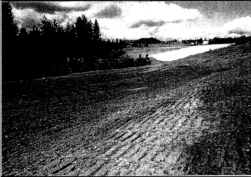
Location 19, looking NW from NE portion of impoundment swale toward dam face, rolling benches in foreground, showing rework from early spring erosion.
