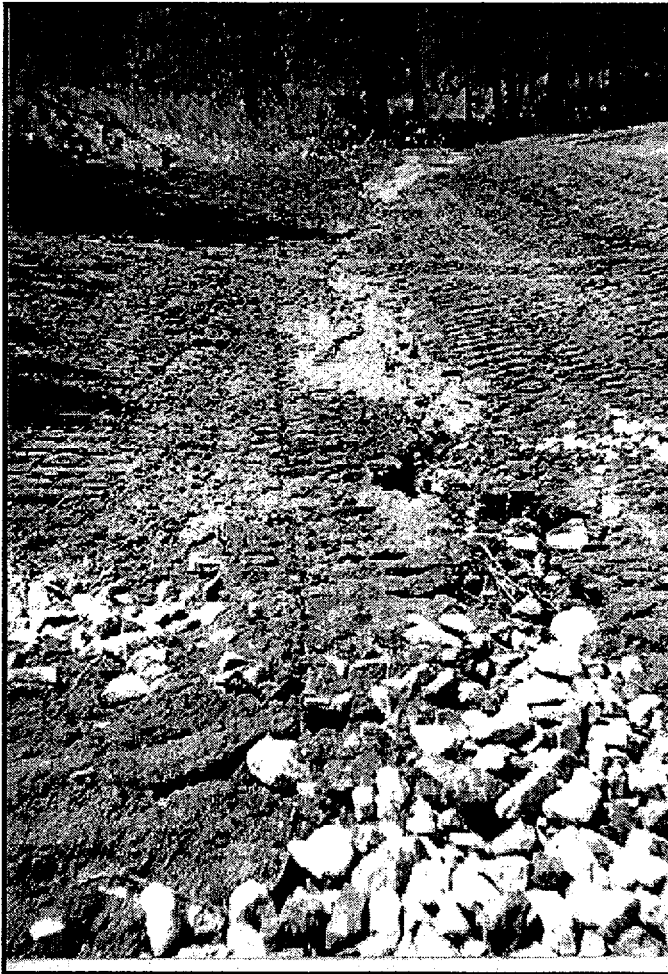
Top: Location 35, looking N from east up slope side of diversion channel showing diversion channel, dike and impoundment in background. Soil lacks fines content, little vegetation.
