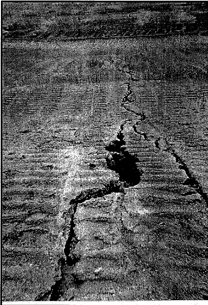
Top: Location 6, looking E from top of margin (down slope), erosion in rills with local depth to 6 inches, erosion starting at slope transition from top of dike, significant vegetation.
