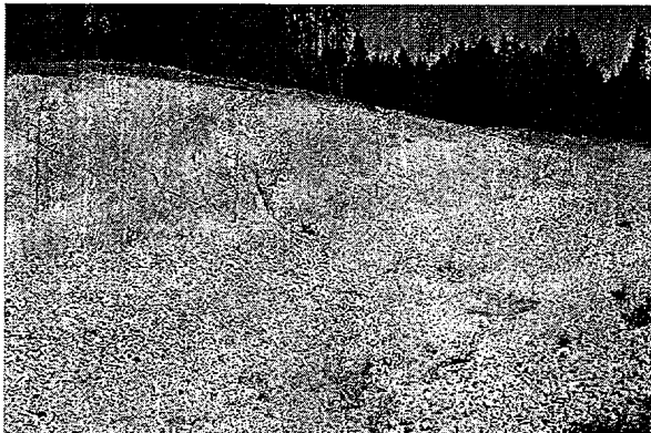
Photograph of the west side of the diversion channel. A sub-soil geological interface has produced a flow concentration effect. This in turn has caused a rill to form and increased soil deposition in the channel at this location.
