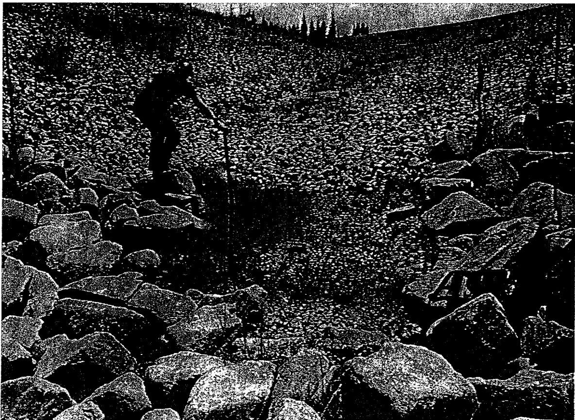
Picture 45: Confluence G downstream transition found void of riprap.
