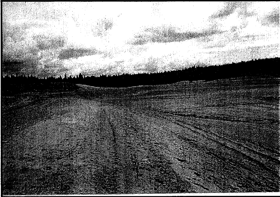
Location 1, looking N from top of dike.
