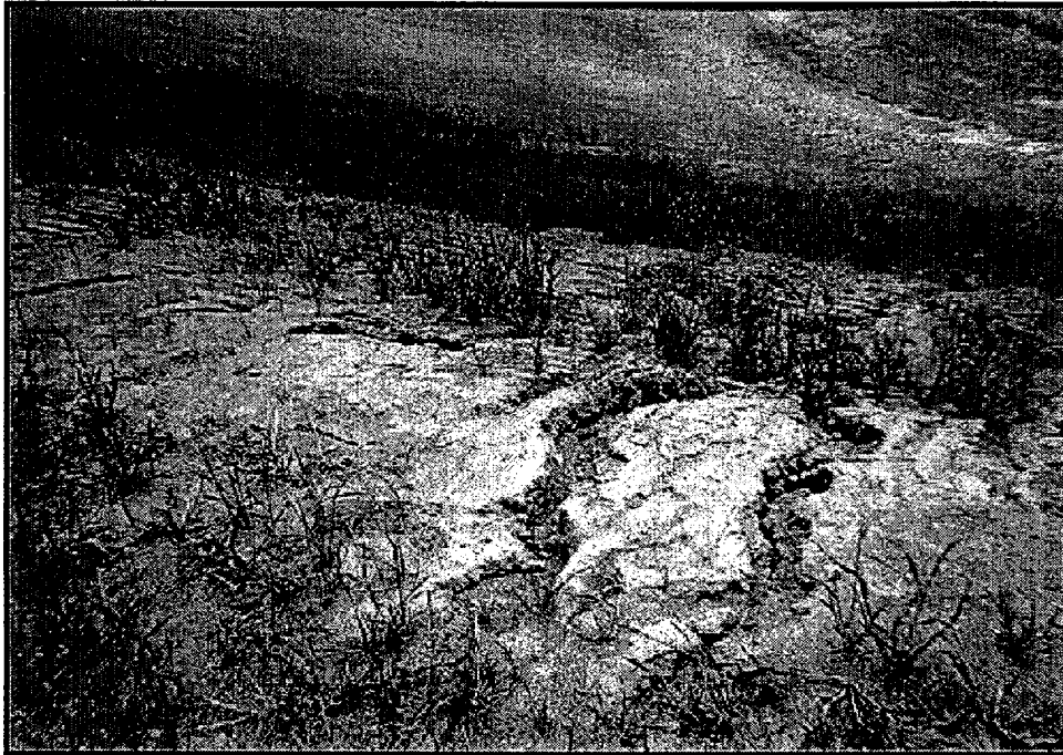
Top: Location 6, looking E from top of margin (down slope), erosion in rills with local depth to 6 inches, erosion starting at slope transition from top of dike, significant vegetation.
