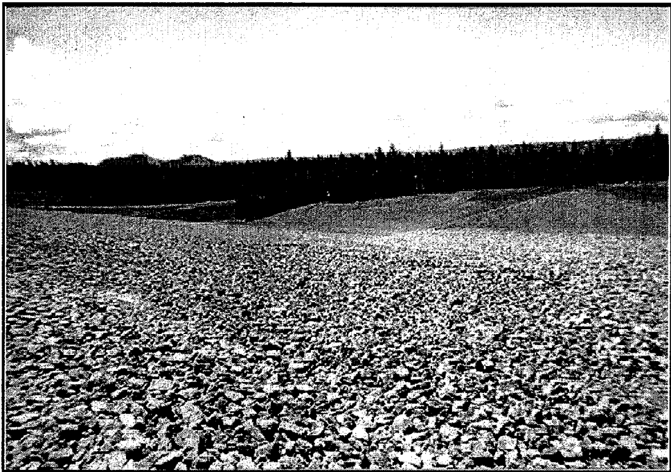
Location 13, looking W S from E end of impoundment dam, dam slope rock erosion protection in foreground, east groin of dam in background.
