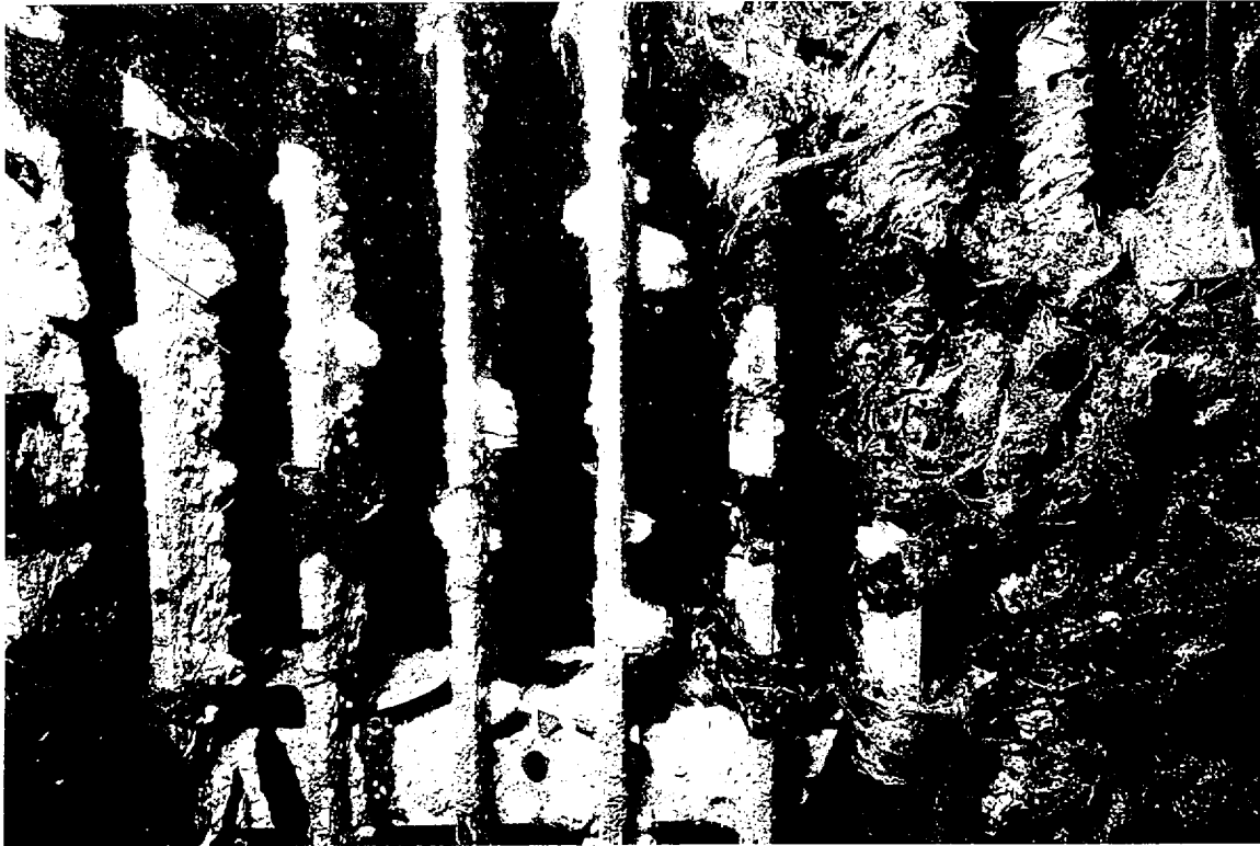
Figure 3-2 Underwater photographs of barnacles and kelp in bar rack openings (upper photograph) and distant view of occluded bar rack openings (lower photograph).
