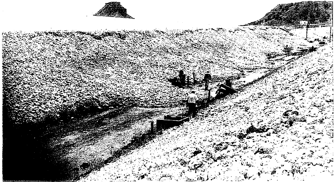
West Slope - Landfill Cell 12 July 15, 1998
