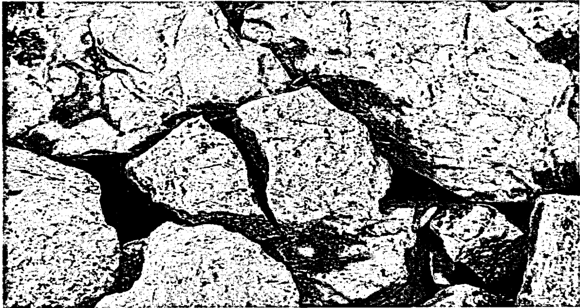
FCT/99. PL-1. Fractured Riprap on Side Slope
