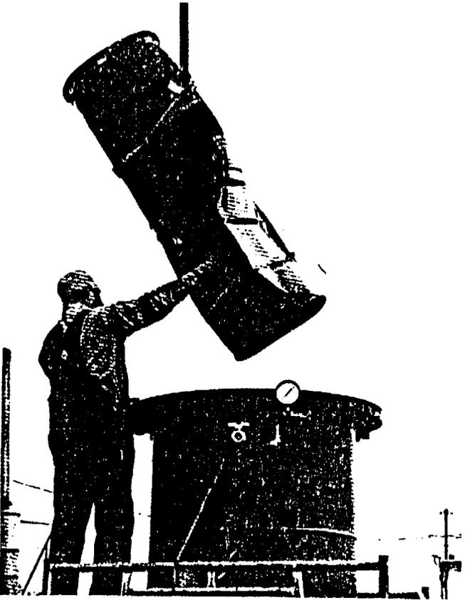
Figure 2.20.2 Removal of Container Following Simulated 15m Immersion Test
