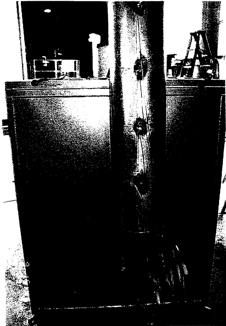
Figure F-2. View of Vessel - Outfitted with Thermocouples.
